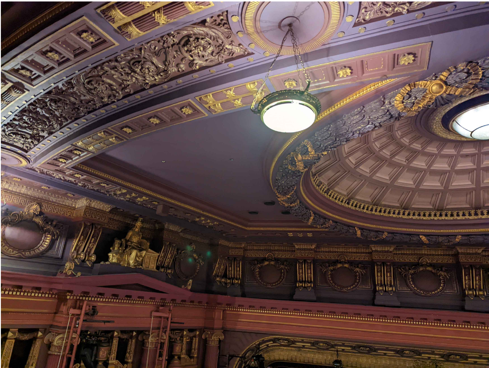
EXISTING AUDITORIUM CEILING PHOTOGRAPH
