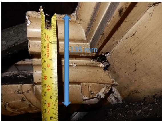
Photos 7 & 8: Showing the depth of a full cast piece that forms the semi-circular rib; and just over half the width of this rib, which are used where these curving ribs terminate the ends of the barrel vault.
