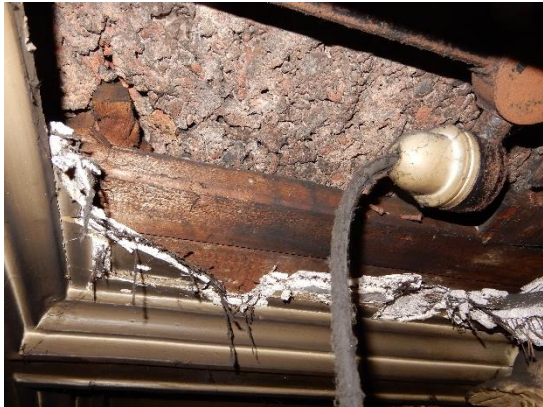
Photos 1, 2 & 3: Early 20 th century steel joists and shuttered concrete carry the floors above the foyers, whose ceilings are hung from a curving timber frame lined with timber boarding.
