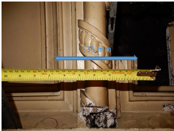
Photo 6: A semi-circular rib across the width
