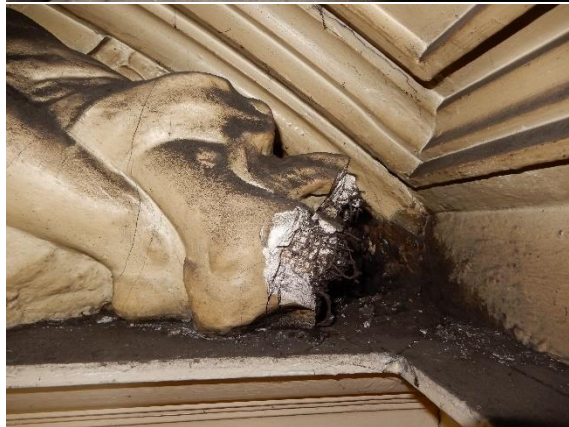
Photos 13-16: Damaged feet on the two figures at entrance No. 75
