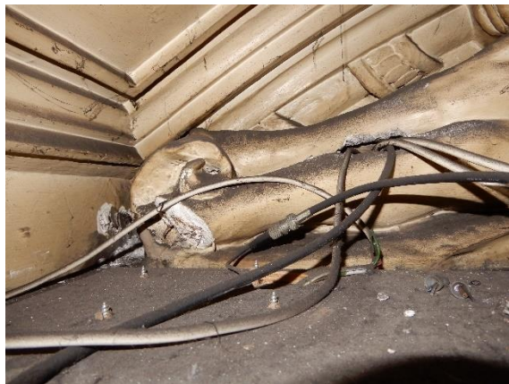
Photos 9-12: Damaged feet on the two figures at entrance No. 73
