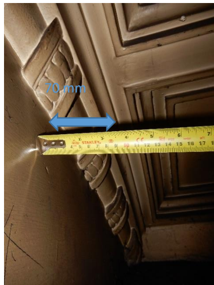
Photos 7 & 8: Showing the depth of a full cast piece that forms the semi-circular rib; and just over half the width of this rib, which are used where these curving ribs terminate the ends of the barrel vault.
