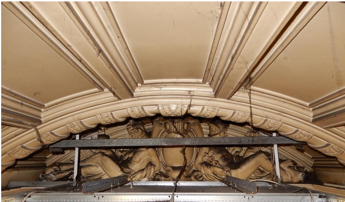
Photo 4: The barrel vaulted ceilings, decorated with plain fibrous cast panels, sub-divided into 15 panels by square ribs, with concave mouldings down their length, and with semi-circular deeper ribs across the ceilings' width, decorated with simple bands. Both are finished with a cartouche and reclining ½ life size classical figures depicting the Greek god Hermes (the Roman Mercury) who was the god of translators and interpreters and ruled over wealth, good fortune, commerce. He carries a ship depicting the trade of goods from India, and opposite a Greek goddess with the world in her hand.
