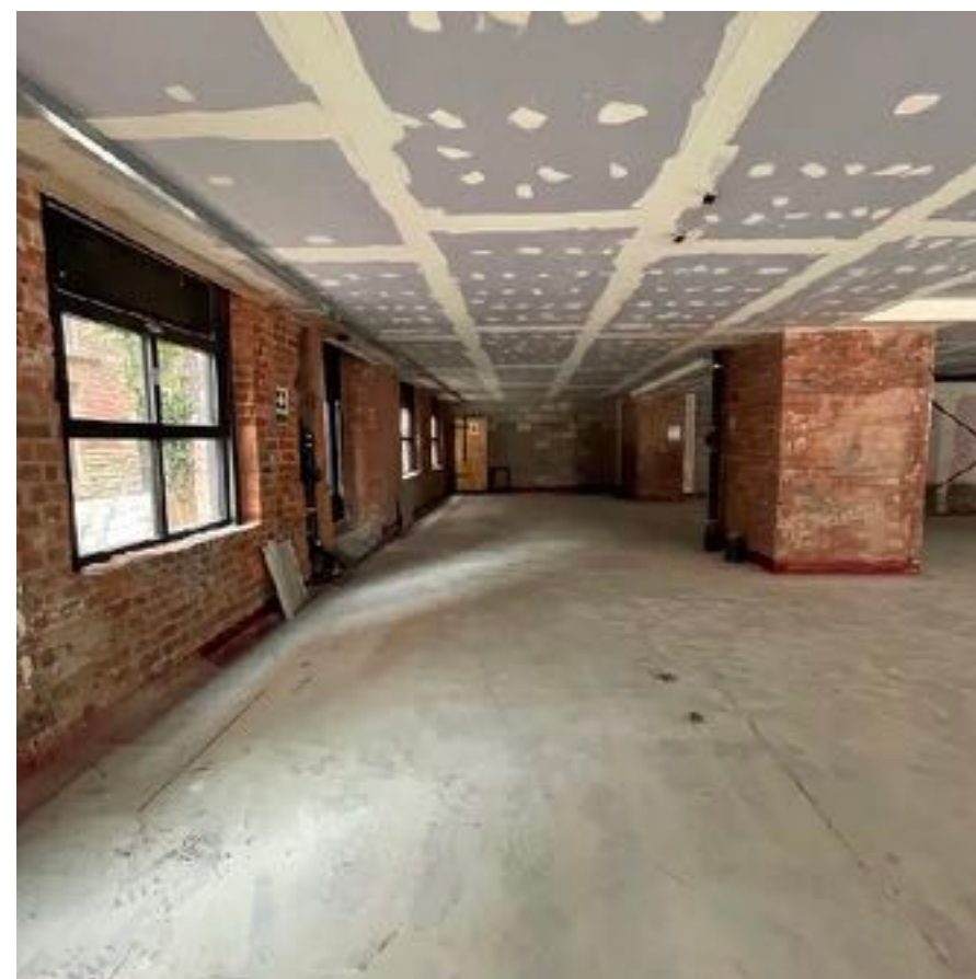
Left wall parallel to Little David Street.
