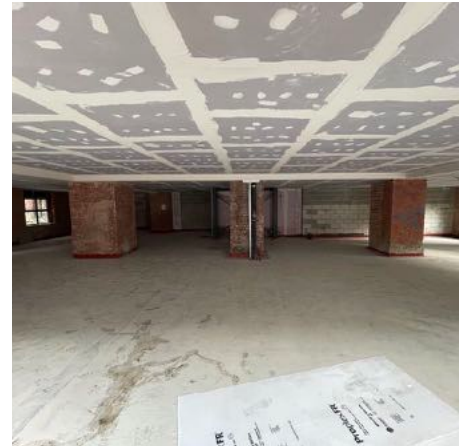
View with back to Chorlton Street.
