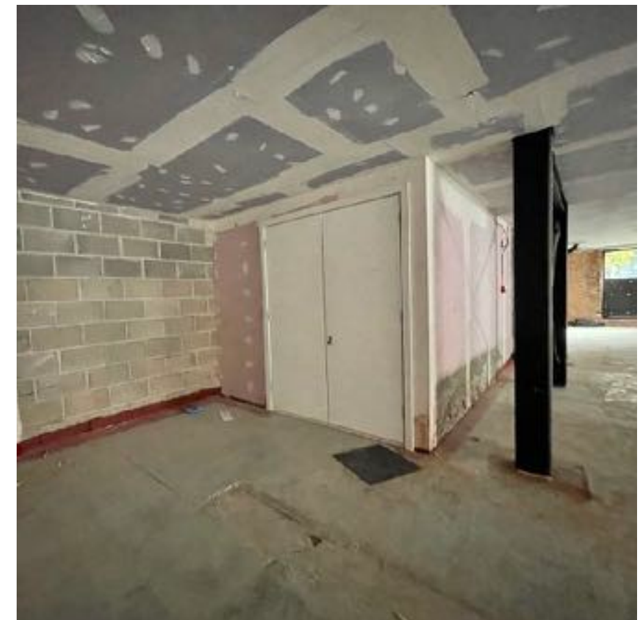
Rear of unit
