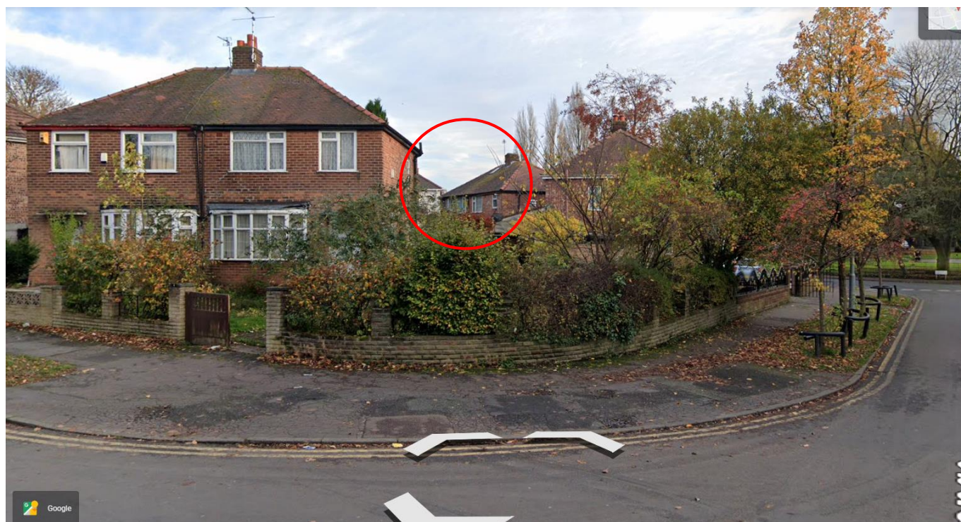
Streetview image showing view of No.11's roof from Crescent Grange
