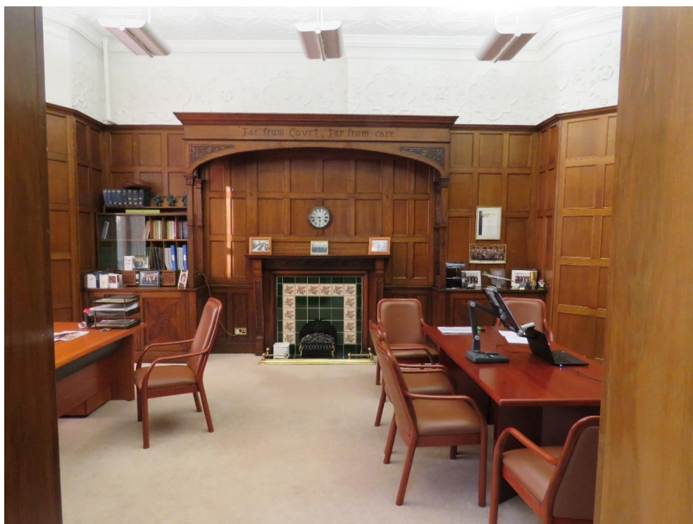
Figure 55 – The north-west reception room, showing the inglenook fire surround and cupboards installed in 1887 – note the decorative frieze to the upper part of the walls and ceiling (see Figure 58). The panelling appears to have been altered/ extended in the 1930s. The inset tiles and fire are modern reproductions.
