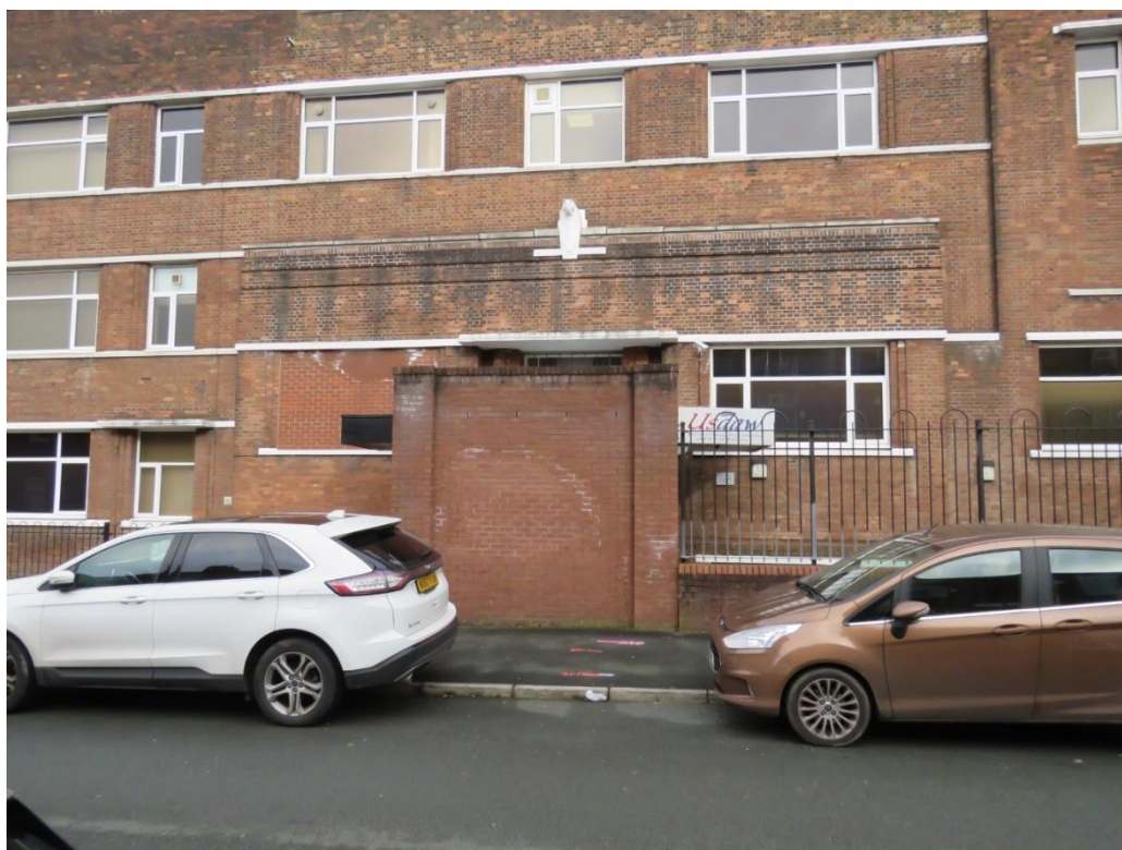
Figure 36 – The 1937 former main entrance on Langley Road which has been blocked off.
