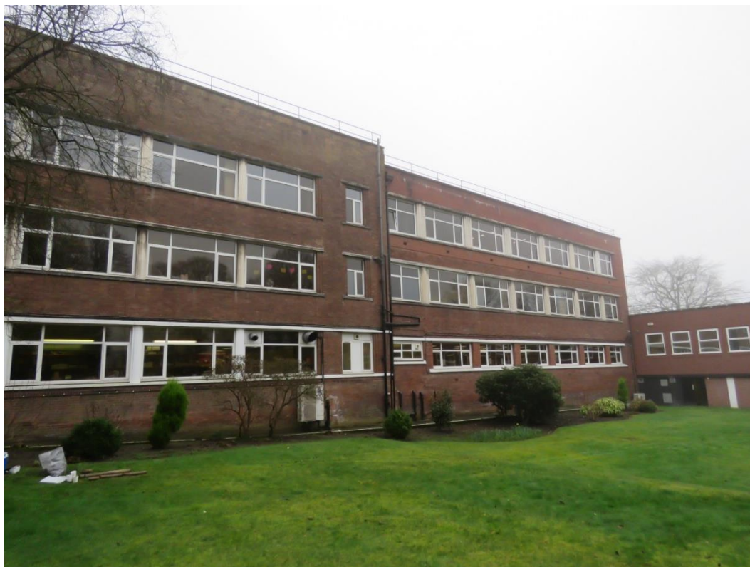
Figure 34 – The north elevation of the 1937 extension (left) and c1950s extension (right).
