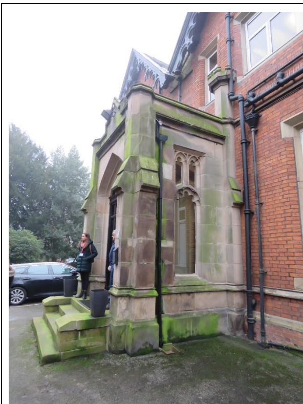
Figure 43 – The original c1837 Gothic entrance porch, showing similar surviving Gothic tracery windows which would have been a feature of the east elevation.
