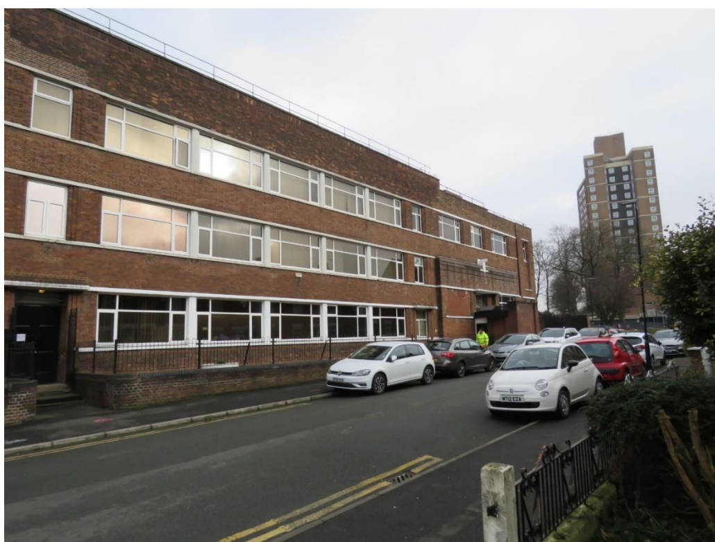
Figure 37 – The Langley Road elevation of the 1937 extension.
