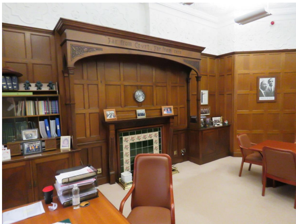
Figure 57 – The 1887 inglenook fire surround, featuring the year “1887” carved into the left and right corner spandrels. The panelling above the cupboards either side of the fire surround dates to the 1930s. The inset tiles are modern reproductions.
