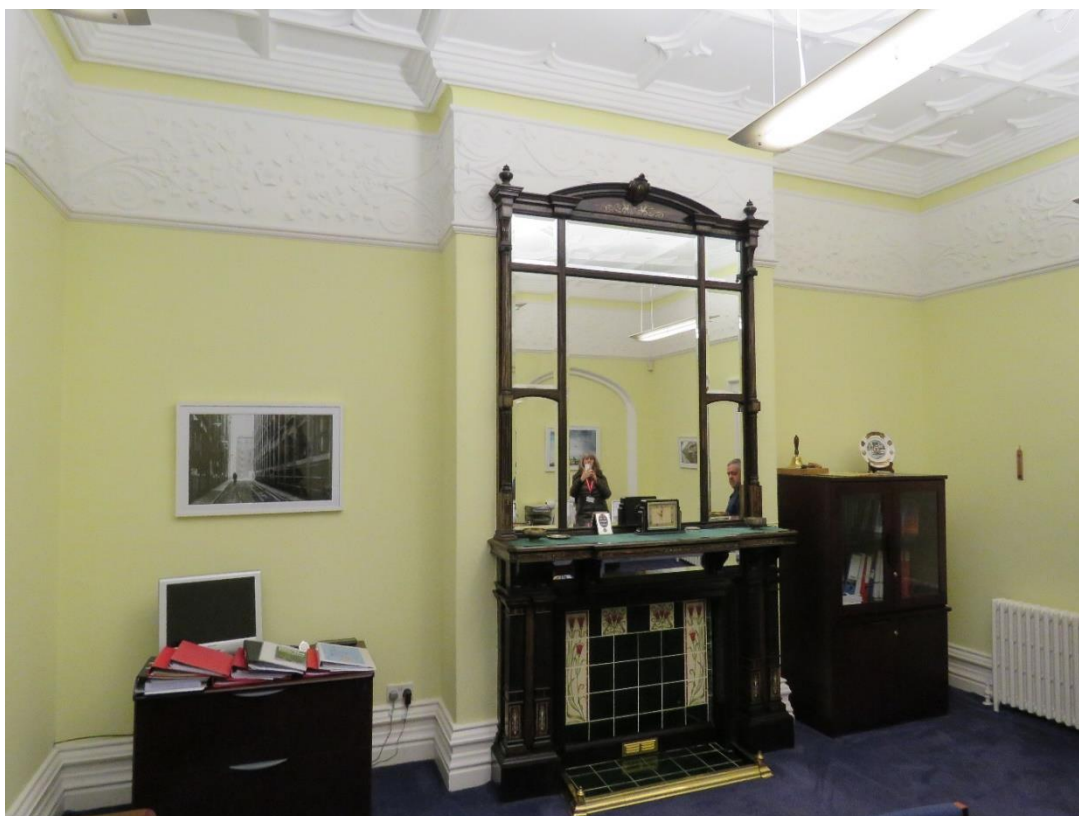
Figure 59 – An original polished slate fire surround and over-mantle mirror to the east elevation of the ground floor, showing original c1837 Gothic ceiling plasterwork, and c1887 plaster frieze.
