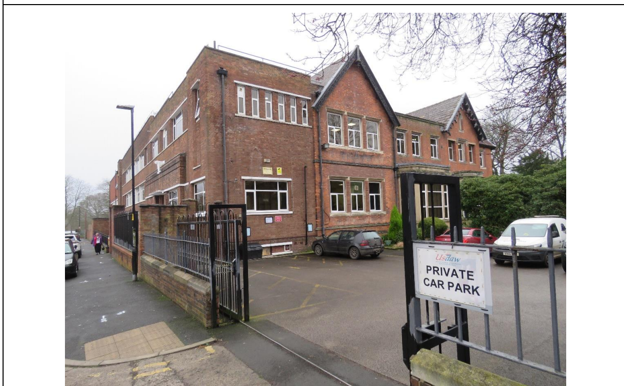
Figure 31 – The east elevation of Oakley (right) showing the 1937 extension to the left. Note the uPVC windows which detract from the appearance of the former house.
