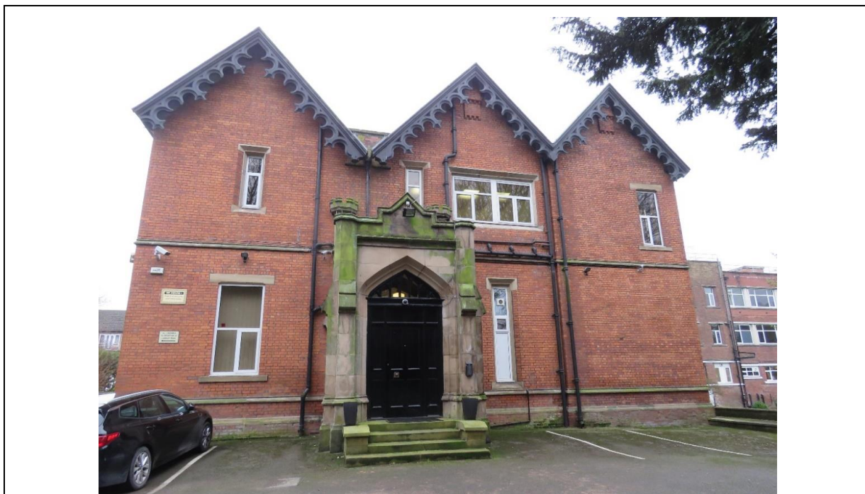
Figure 30 – The original entrance to the north elevation. Note the uPVC windows which detract from the appearance of the former house.
