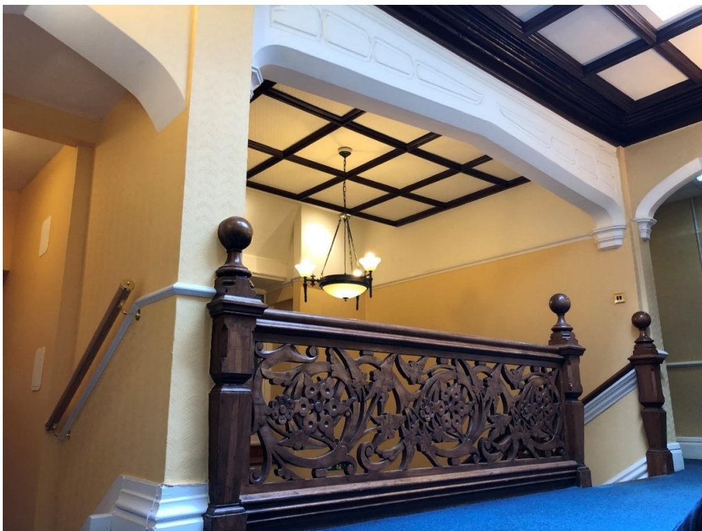
Figure 62 – The first floor landing, showing the c 1880s carved timber balustrade.
