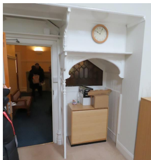
Figure 52 – The inside face of the internal window, which appears to have been inserted in the c1880s.
