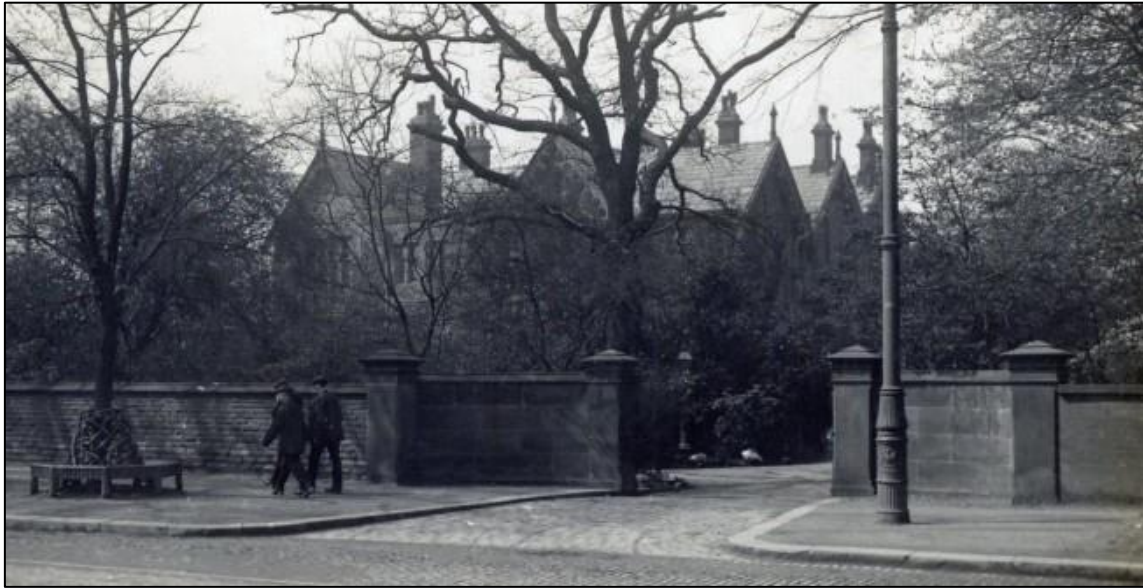
Figure 6 – View c1900. Photograph above is of 'Oakley', one of the three large mansions built on the western side of Fallowfield Brow in the early 19th century.
