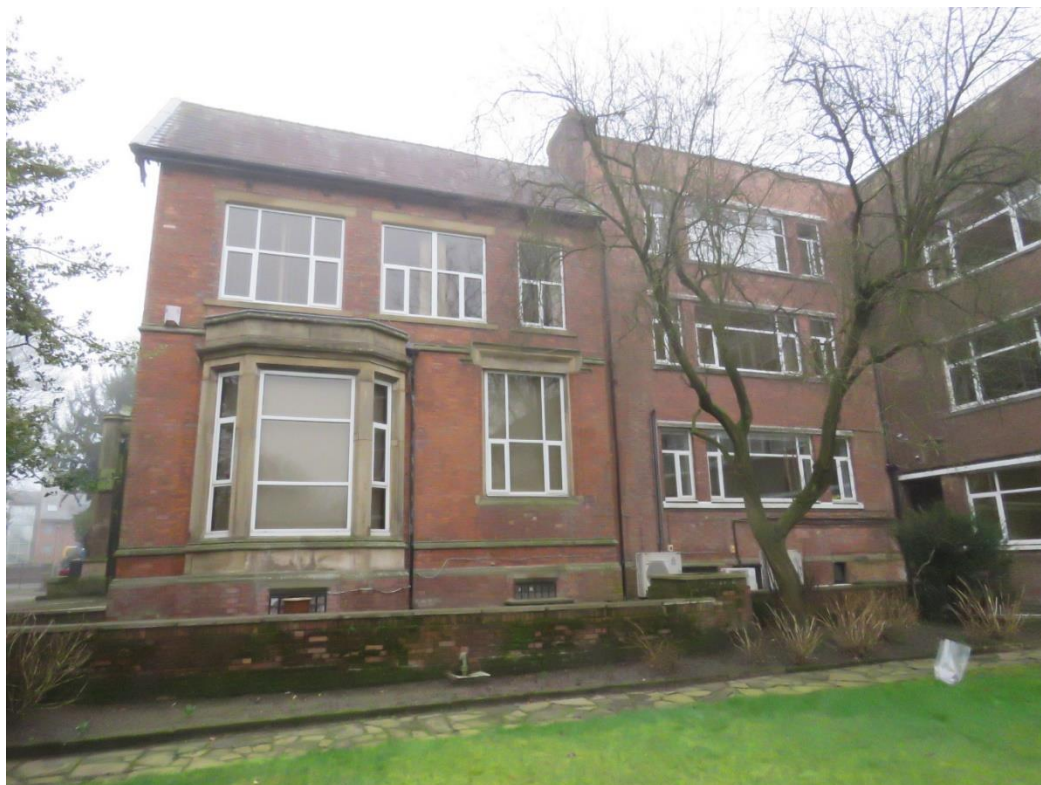
Figure 32 – The west elevation. Note the insertion of uPVC windows which detracts from the appearance of the house.
