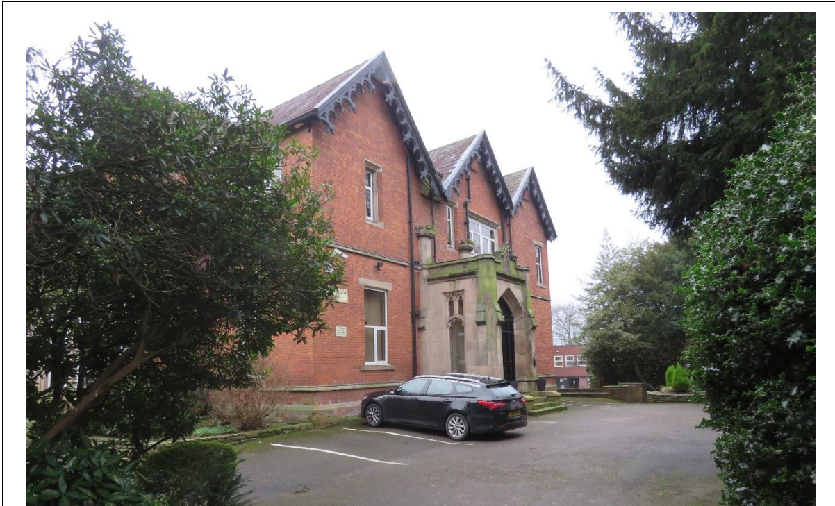
Figure 2 – The principal entrance front of the early-19 th century villa.
