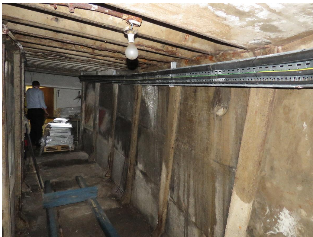
Figure 69 – possible access tunnel/ ventilation passage (see Figure 22) possibly modified for Air Raid Protection measures in the 1940s.
