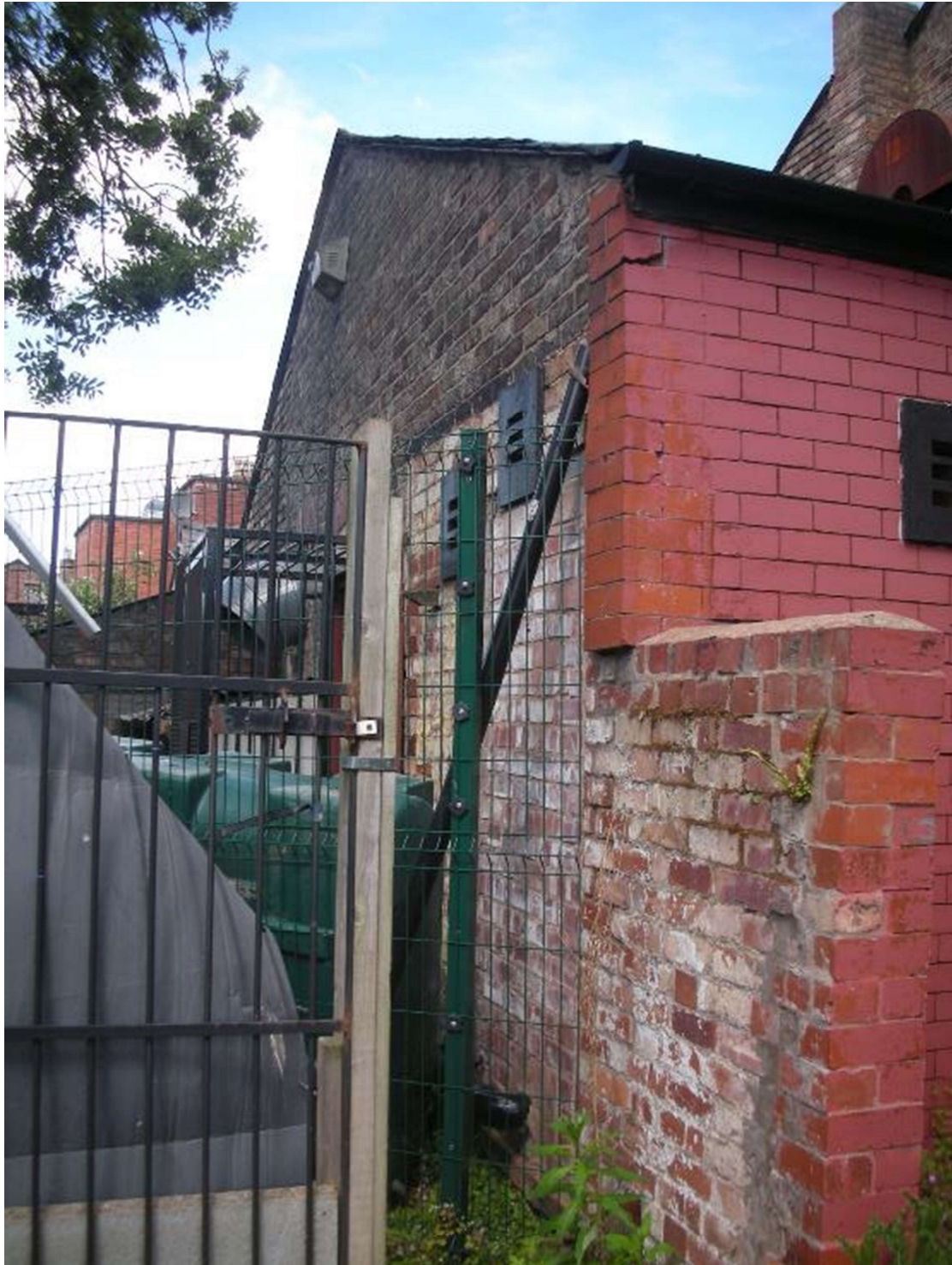
Figure 11: Demolished outbuilding (white outline on wall)
