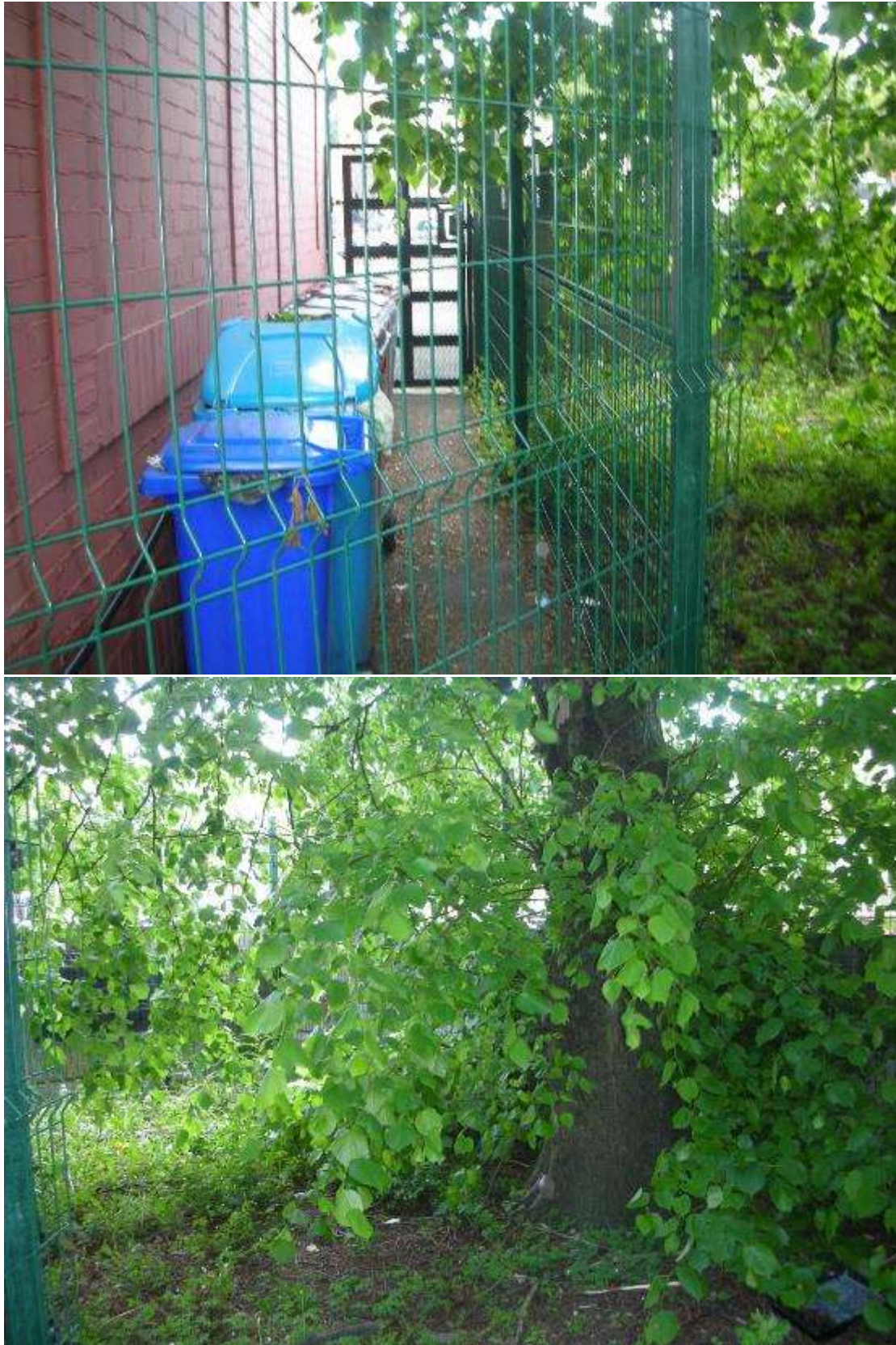
Figure 16: Eastern boundary and access gate from Withington Road
