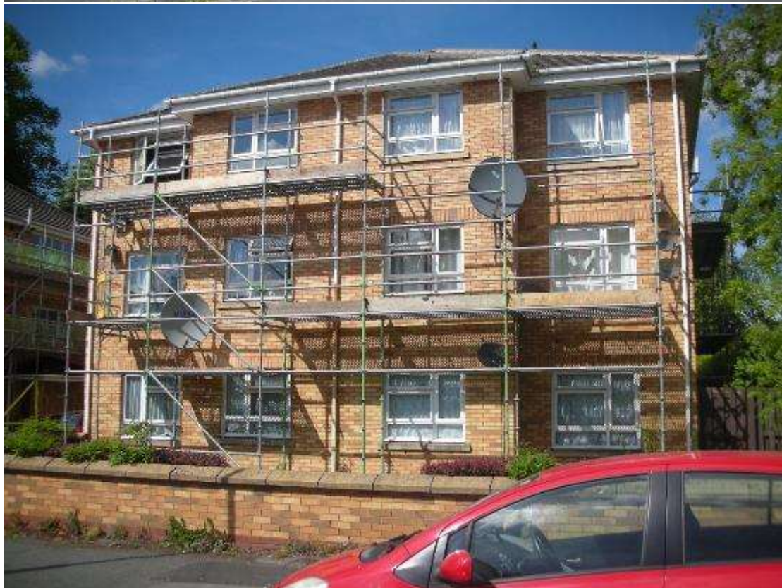
Figure 21: Further Views from the street of site and number 2
