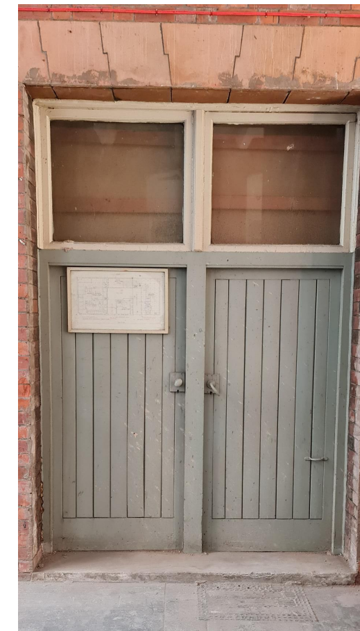
Photograph of Existing Door 28/03/22
