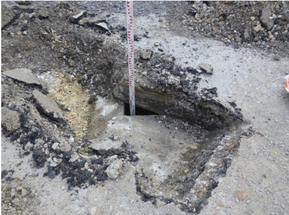
Figure 3-2-Abandoned chamber found during GI
