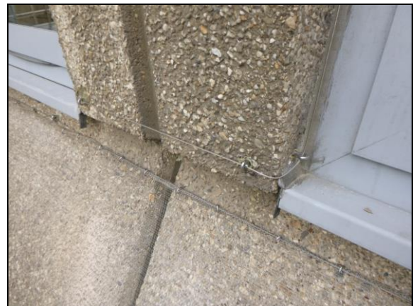
Figure 6: Example of netting installation.
