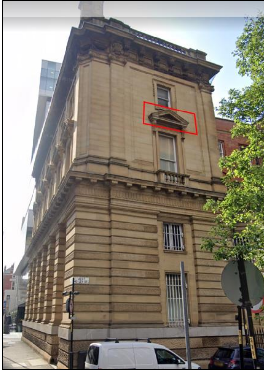
Figure 3: Image showing extent of proposed pigeon netting installation – West Mosley Street.
