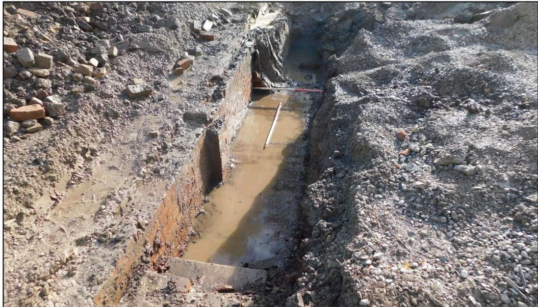
Plate 3: Trench 3 looking southeast
