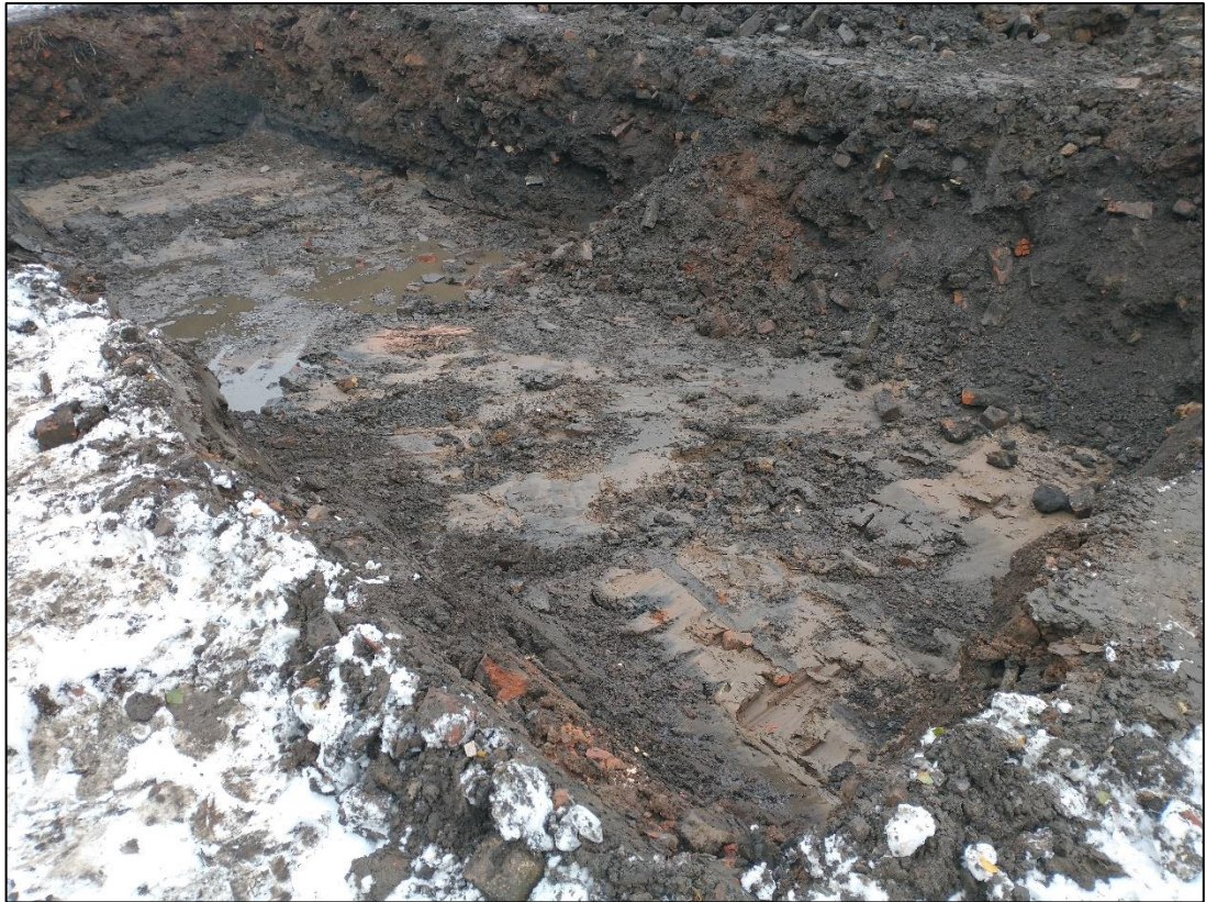
Plate 6: Excavation area A1 looking north
