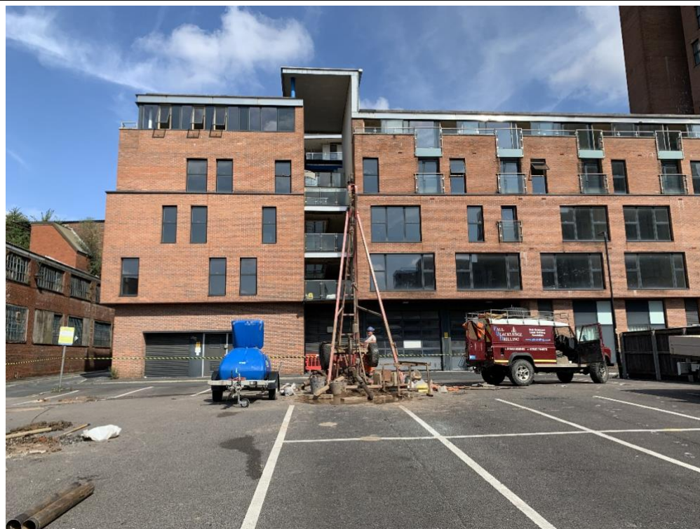
Figure 3 View Facing Northwest Showing the Cable Drilling in the Northern Portion of the Site
