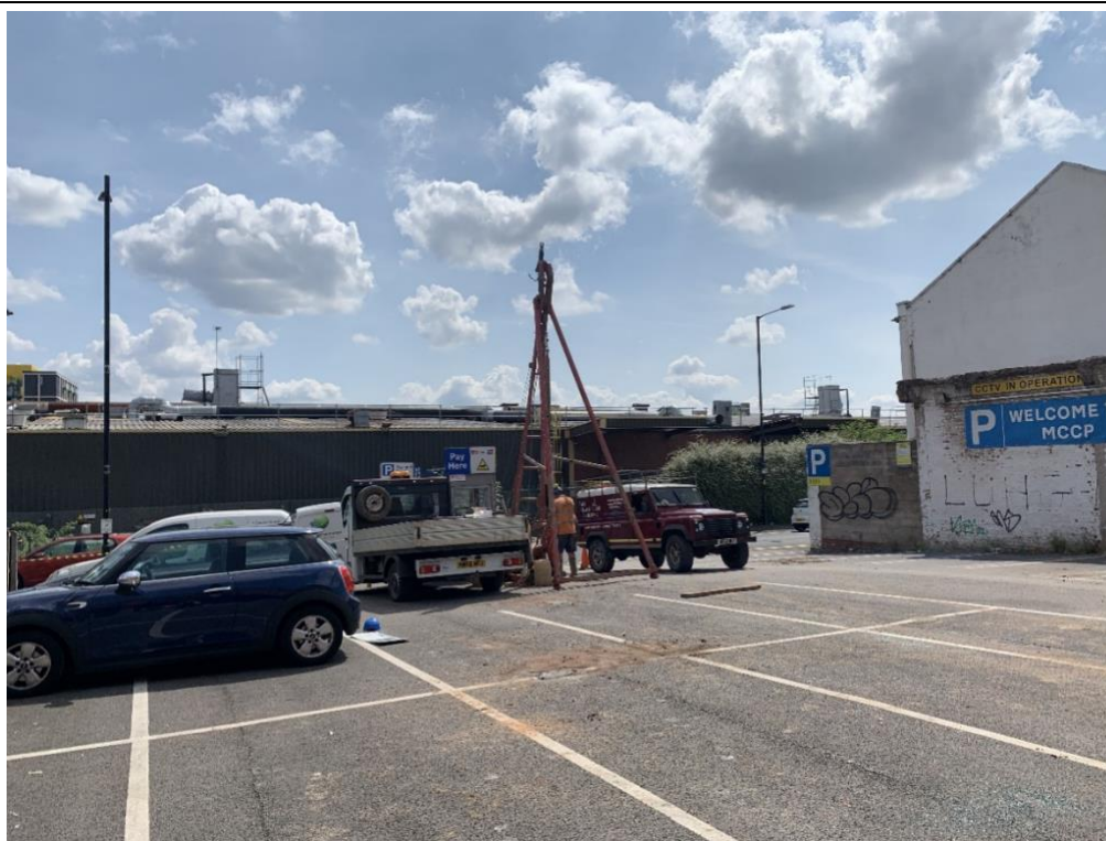
Figure 4 View Facing Southeast Showing the Cable Drilling in the Southern Portion of the Site
