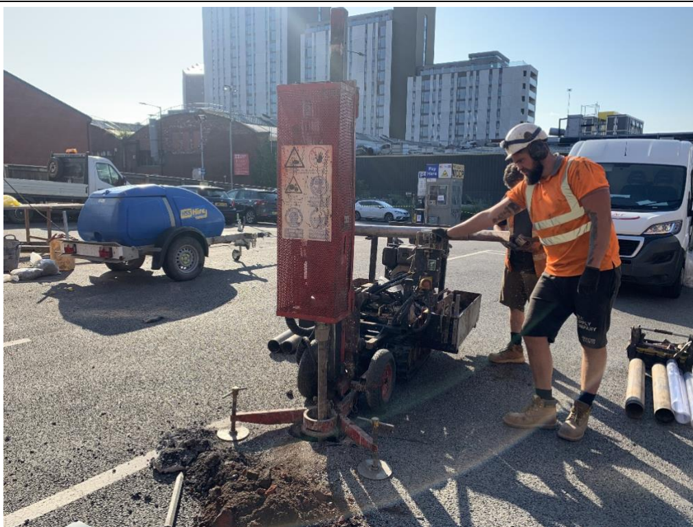
Figure 2 View Facing Southeast Showing the Window Sampling Setup
