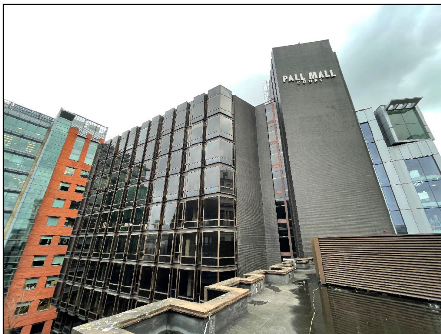
Photograph A2.4: View from western roof, on fifth floor, looking back at the central Pall Mall building
