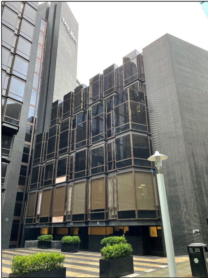
Photograph A2.3: Pall Mall from ground-level, with central column in background.
