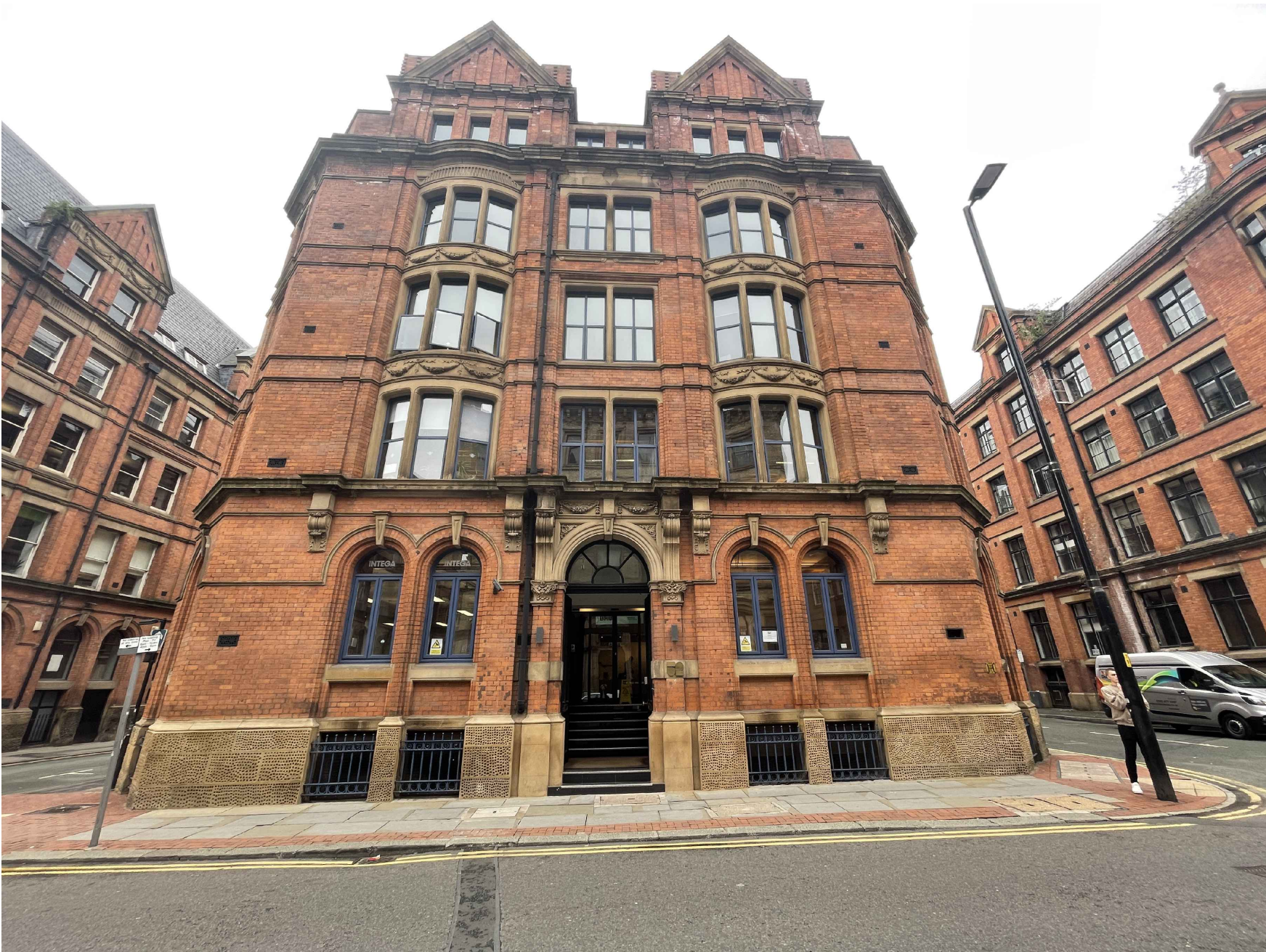
EXISTING IMAGE OF FRONT FACADE
