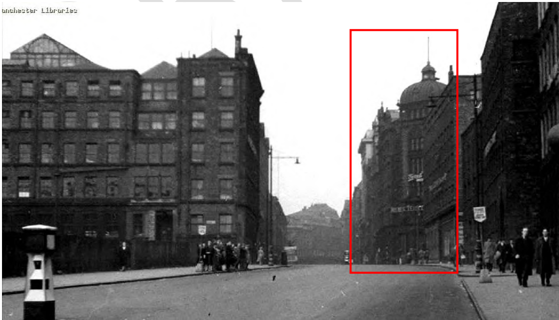
Figure 55: 1960 – Looking east up Cannon Street towards its continuation into Church Street and the junction with High Street, showing the cleared north side of Cannon Street and the elaborate corner tower of Holmes, Terry & Company's Edwardian building.
