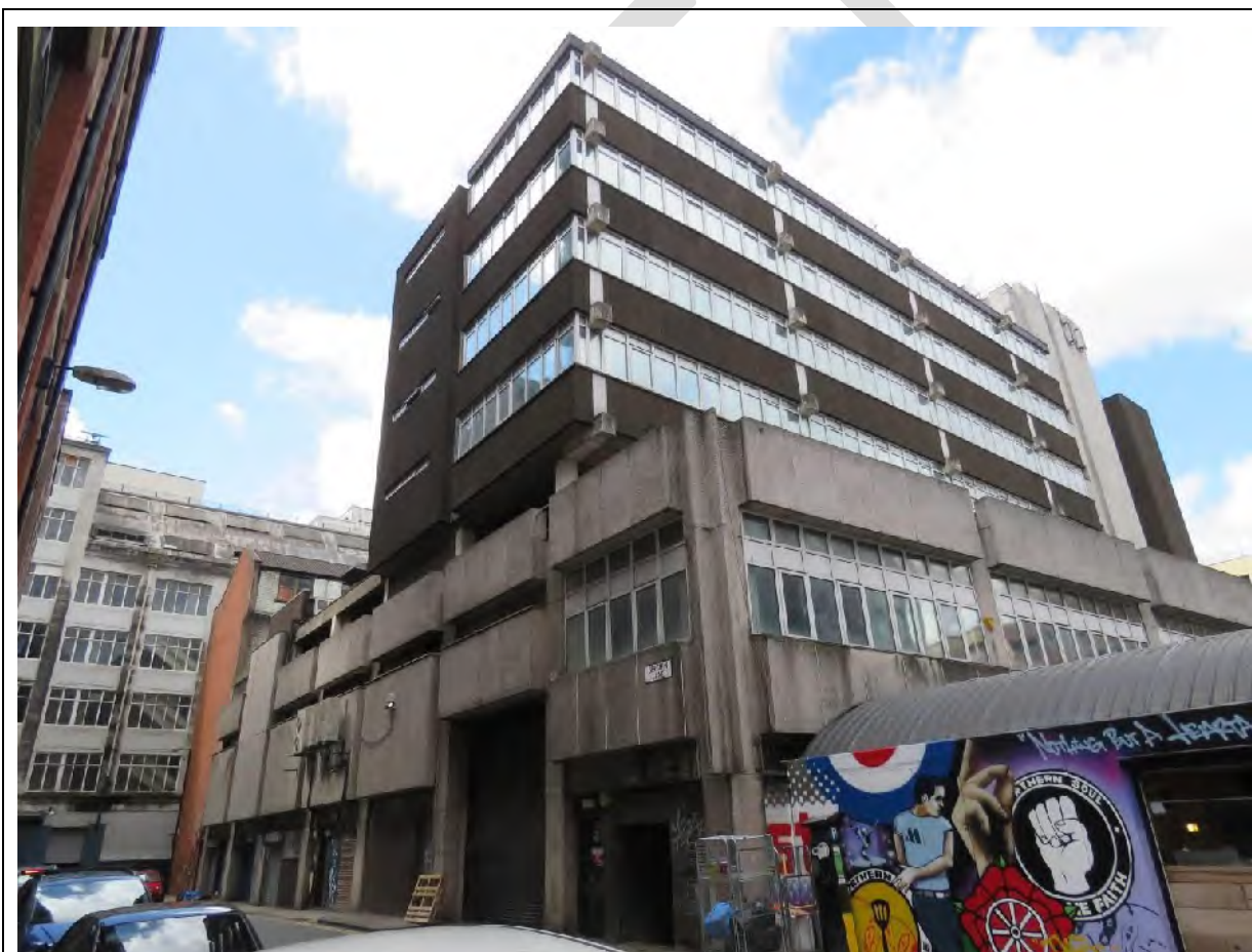
Figure 63: The rear Birchlin Street (east) elevation in 2017
