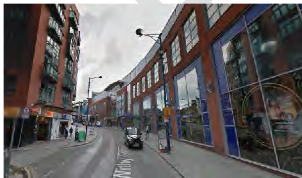
Figure 73: Looking east along the curved Withy Grove, showing the northern side of the Arndale Centre to the right. The historic character within this view has been eroded.
