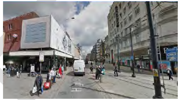
Figure 72: Looking north along High Street from its junction with Market Street. There is no consistency to the character of this view as it is a mix of different types, form, styles and dates of buildings
