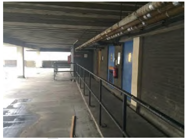
Figure 67: The covered car deck and access into the building.
