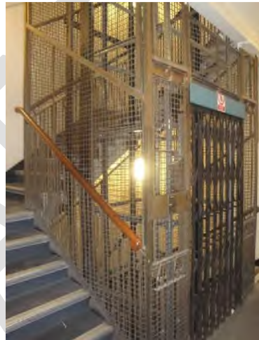
Figure 36: The original cage lift and staircase with altered lift.
