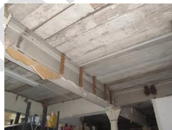
Figure 44: The exposed original ceiling structure and columns on the upper floors.
