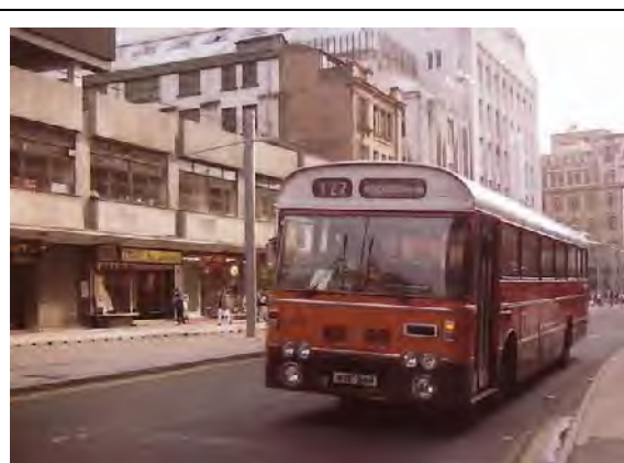
Figure 62: 1991 – A view looking south down High Street from outside the Arndale Centre, showing the original shop fronts and windows.
