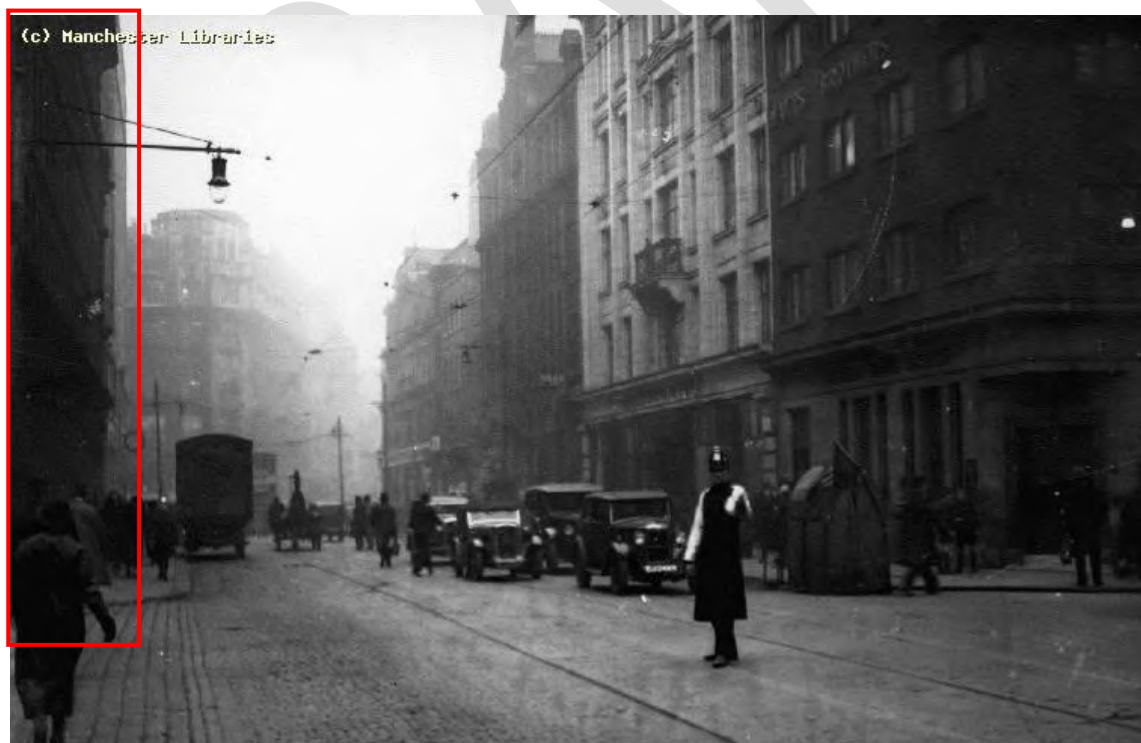
Figure 58: 1930 – Looking south along High Street towards Lewis's Department Store (now Primark). The subject site can be glimpsed to the left of the image.
