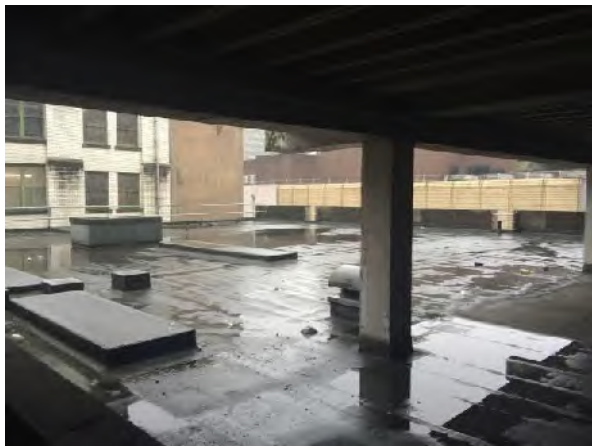
Figure 66: The covered car deck at second floor level, looking towards the white glazed brick former loading court of No. 20-22.
