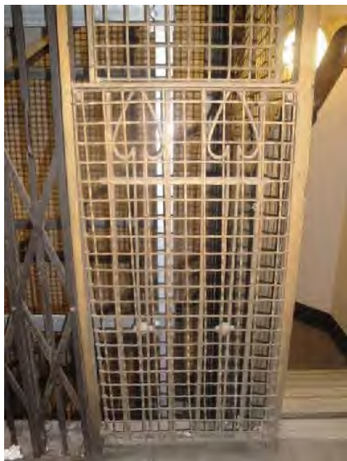
Figure 37: Detail of the Art Nouveau cage lift decoration.
