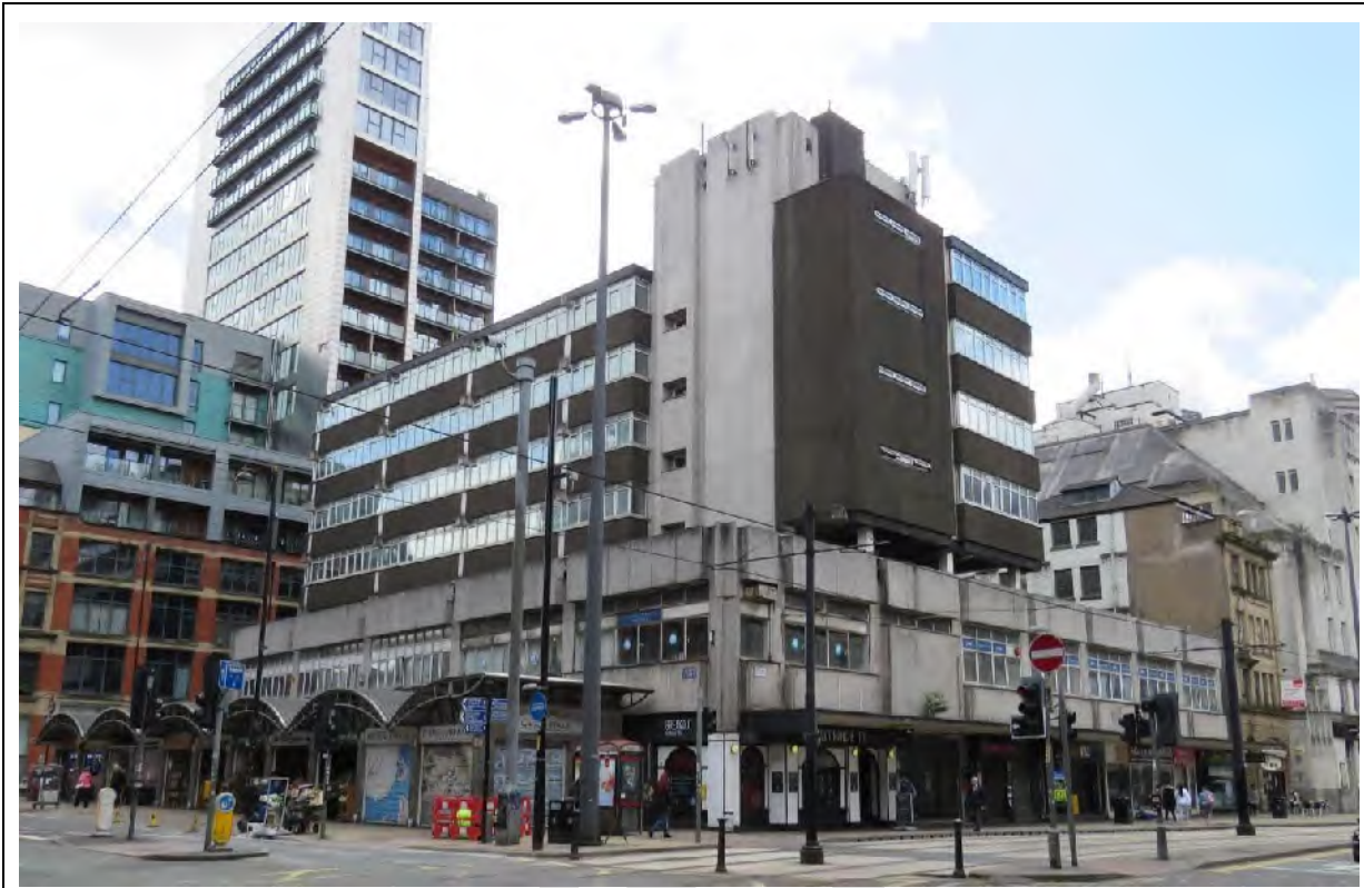
Figure 51: The Church Street (north) and High Street (west) elevations of 24-36 High Street in 2017.
