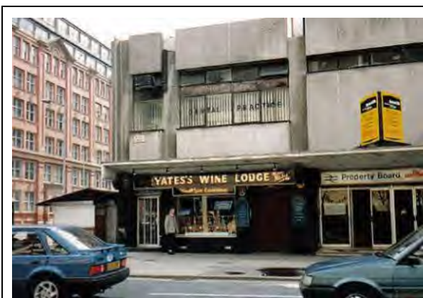
Figure 61: 1990 – A view of the corner of High Street and Church Street showing the original metal framed windows which have now largely been replaced with UPVC.
