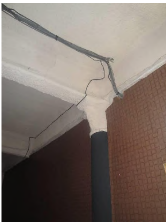
Figure 41: A detail of the cast iron columns which can be found on each warehouse floor.
