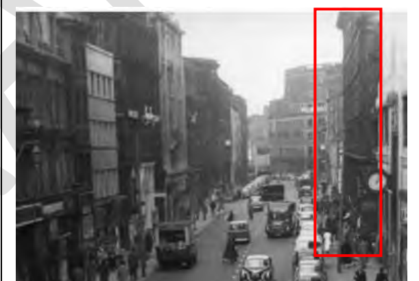
Figure 21: 1951 – The same view in 1951 showing the 1929-32 new Ryland's building (now Debenhams) to the right, and the subject site beyond.
