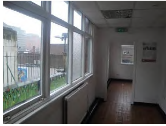
Figure 46: The top floor which is located within the roof structure, looking out onto the southern terrace which extends around the south and west of the building.
