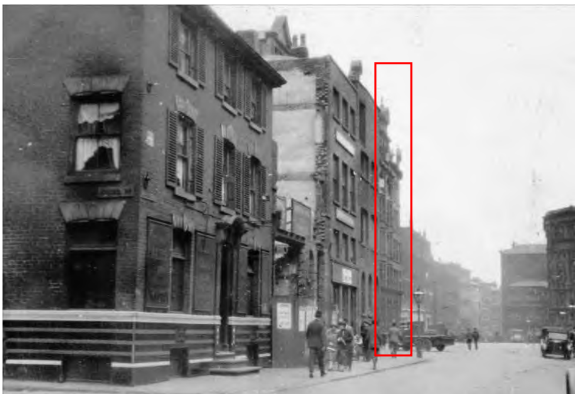
Figure 57: 1925 – Looking west along Church Street during a later phase of demolitions and road widening to the southern side of the street. Note the already rebuilt corner of the subject site circled in red.
