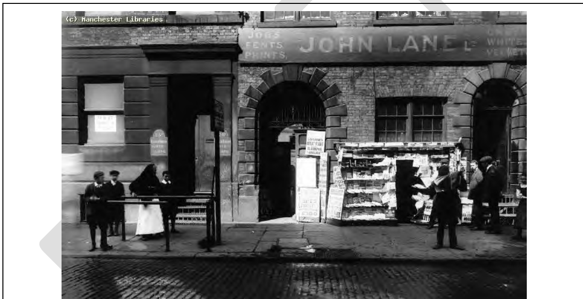
Figure 4: A view looking across at the original buildings on the western side of High Street, as seen from the subject site in 1910. This view illustrates the differing early building types found in the area during the 1900s.
