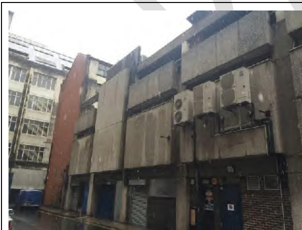
Figure 64: The east (rear) elevation of the building, showing the 1989 reconstructed red brick rear elevation of No 20-22 High Street to the right.
