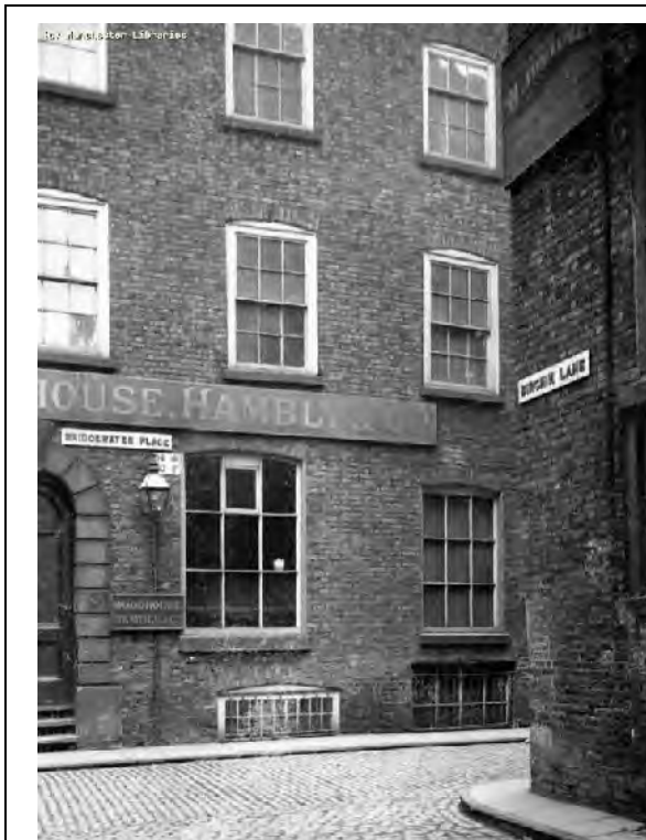
Figure 16: 1900 – The corner of Bridgewater Place and Birchin Lane looking south towards the early-19 th century extension of the former Bridgewater Arms. Note the rear elevation of the original building on the site of 20-22- High Street to the right.
