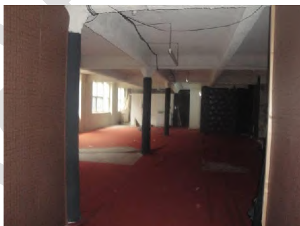
Figure 40: The first floor warehouse floor looking east showing the north windows which originally looked onto the loading court.
