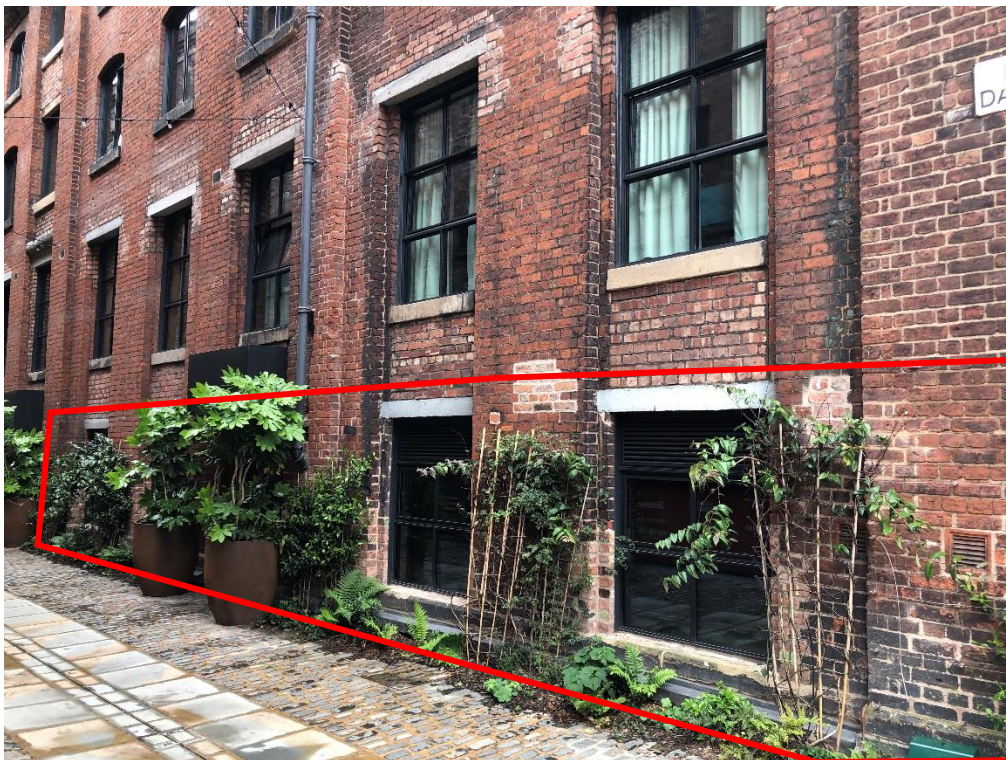
Figure 6: The Little David Street (north-west) elevation of the unit (outlined), showing two of its windows and a third entrance door concealed by planning to the left.
