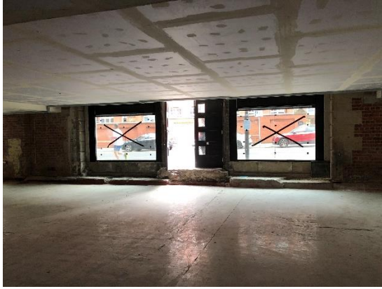
Figure 7: Looking south-west through the unit towards the entrance from Chorlton Street, showing the modern dropped ceiling and modern concrete floor.
