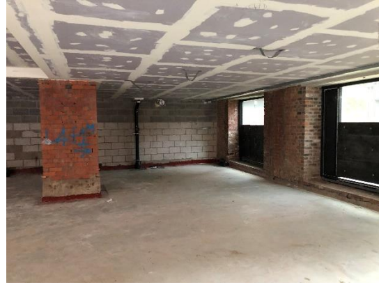
Figure 8: Looking north-east through the unit towards the south-west elevation/modern window openings, showing the modern dropped ceiling, modern concrete floor, and modern blockwork wall to the rear. Note one of the three original brick piers to the left.
