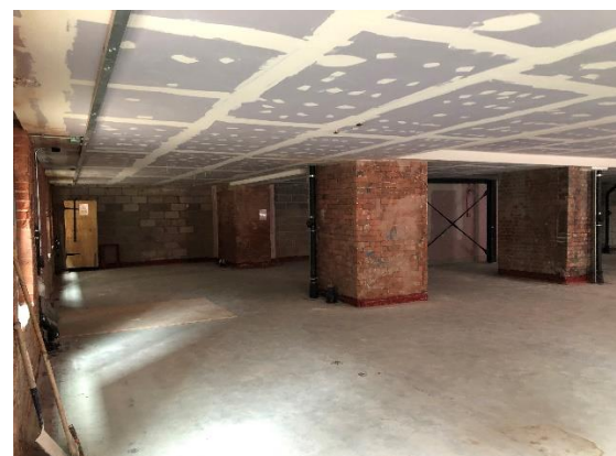
Figure 12: Looking east along the north-west elevation (left) showing the modern blockwork to the rear of the unit, which can be seen to partly conceal the northernmost brick pier.
