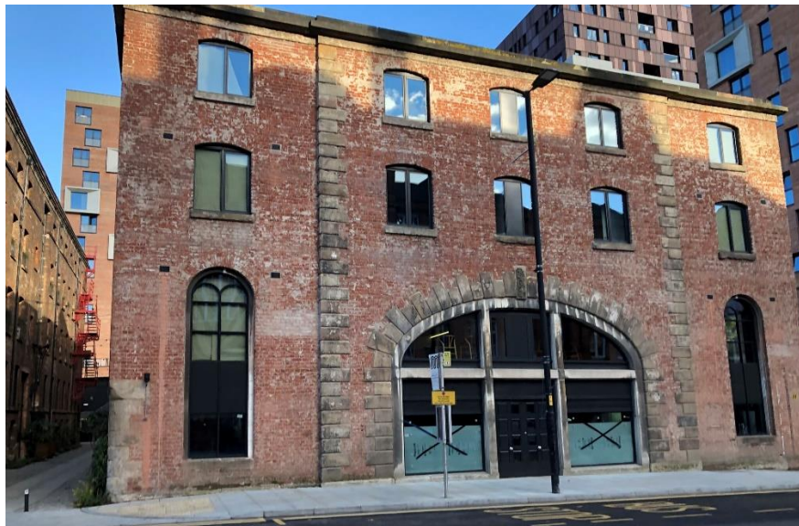
Figure 2: The completed principal elevation of Minshull House as seen from Chorlton Street in 2022, the ground floor level of which contains the proposed MADRE unit.
