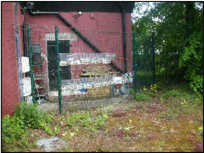
Fencing from 120A
