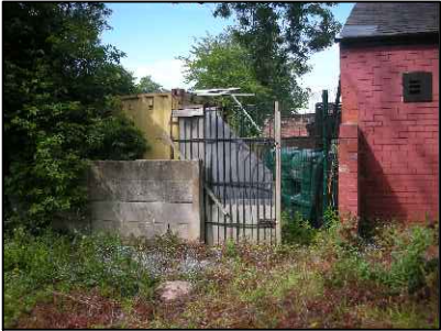
Demolished outbuilding location
