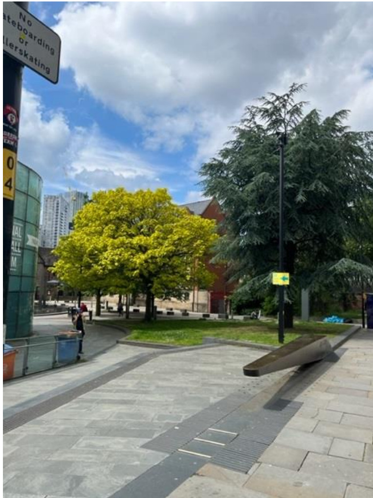
Figure 2- Column Mounted CCTV Camera 1 location
