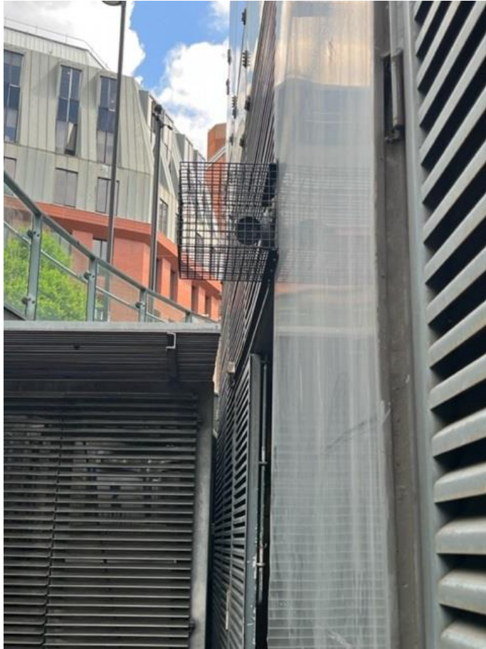
Figure 4- Building Mounted CCTV Camera 2 location
