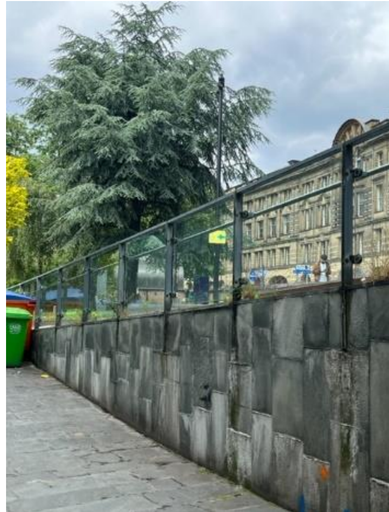
Figure 3- CCTV Camera 1 viewed from external ramp location.
