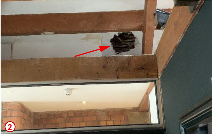
REMEDIAL WORKS TO SLANTED PLASTERED CEILINGS
