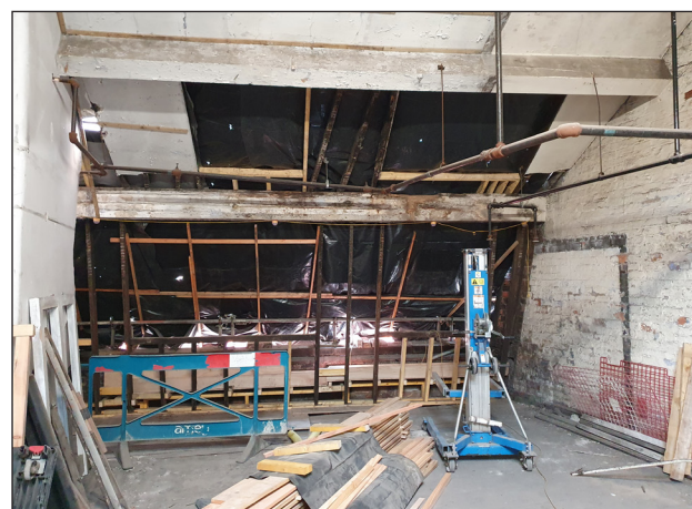
IMAGE 11: Internal Photo - Fourth Floor Breakout Space
