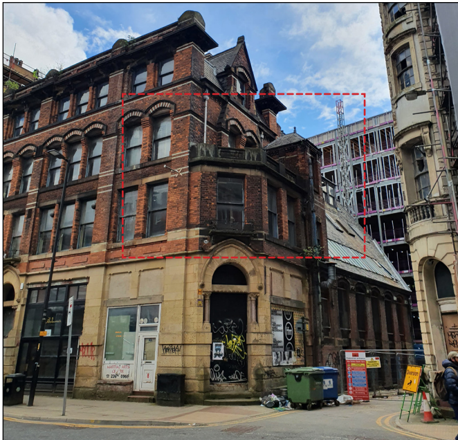
IMAGE 5: External Photo of Existing Roof to Form the External Terrace - Second Floor Breakout Space
