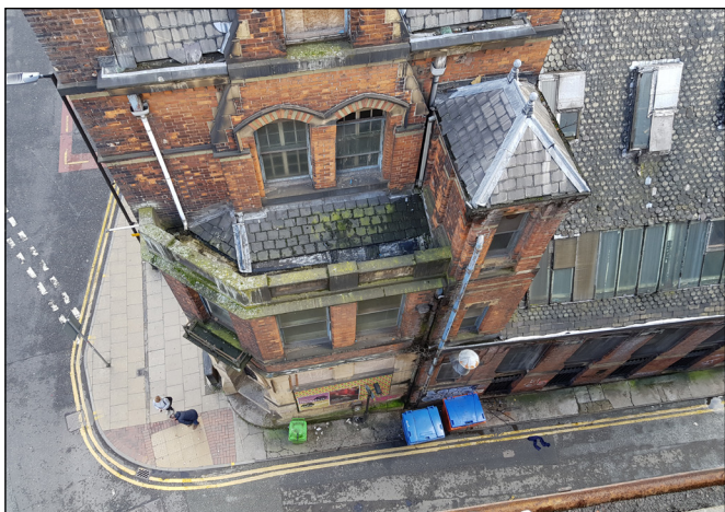
IMAGE 6: Existing Aerial View - Second Floor Breakout Space
