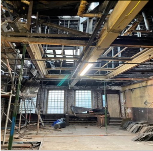
upper floor floor number 12 post removal of ceiling
