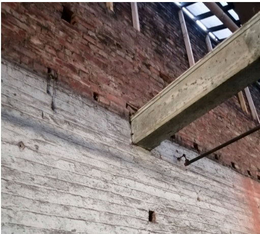
detail of wall showing paint and brickwork where ceiling once were and in addition sockets for ceiling joists. These features will remain.
