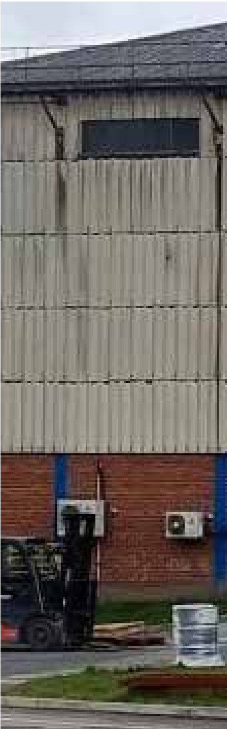
Existing North Facade
