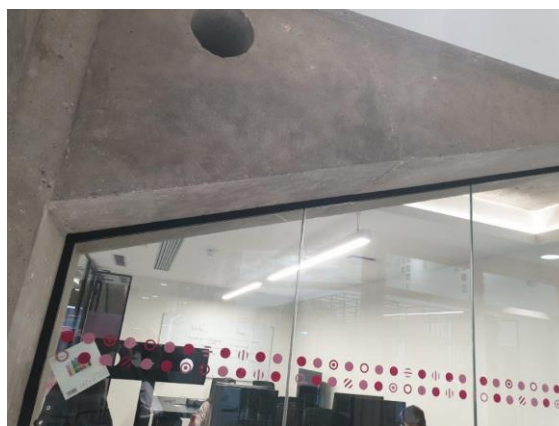
Image 10: Ground floor. Glazed partition abutment.
