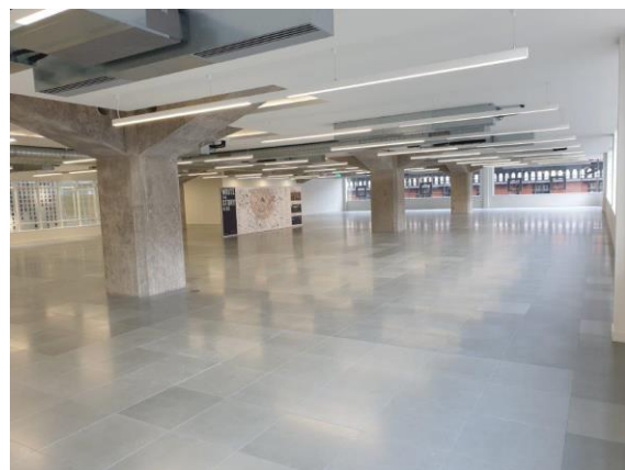
Image 4: 2 nd floor interior
