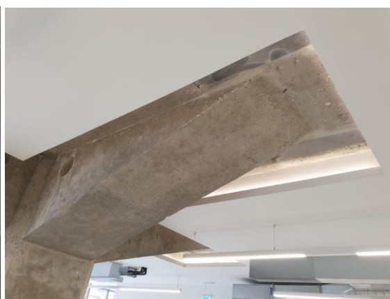
Image 6: Underside of cruciform concrete column
