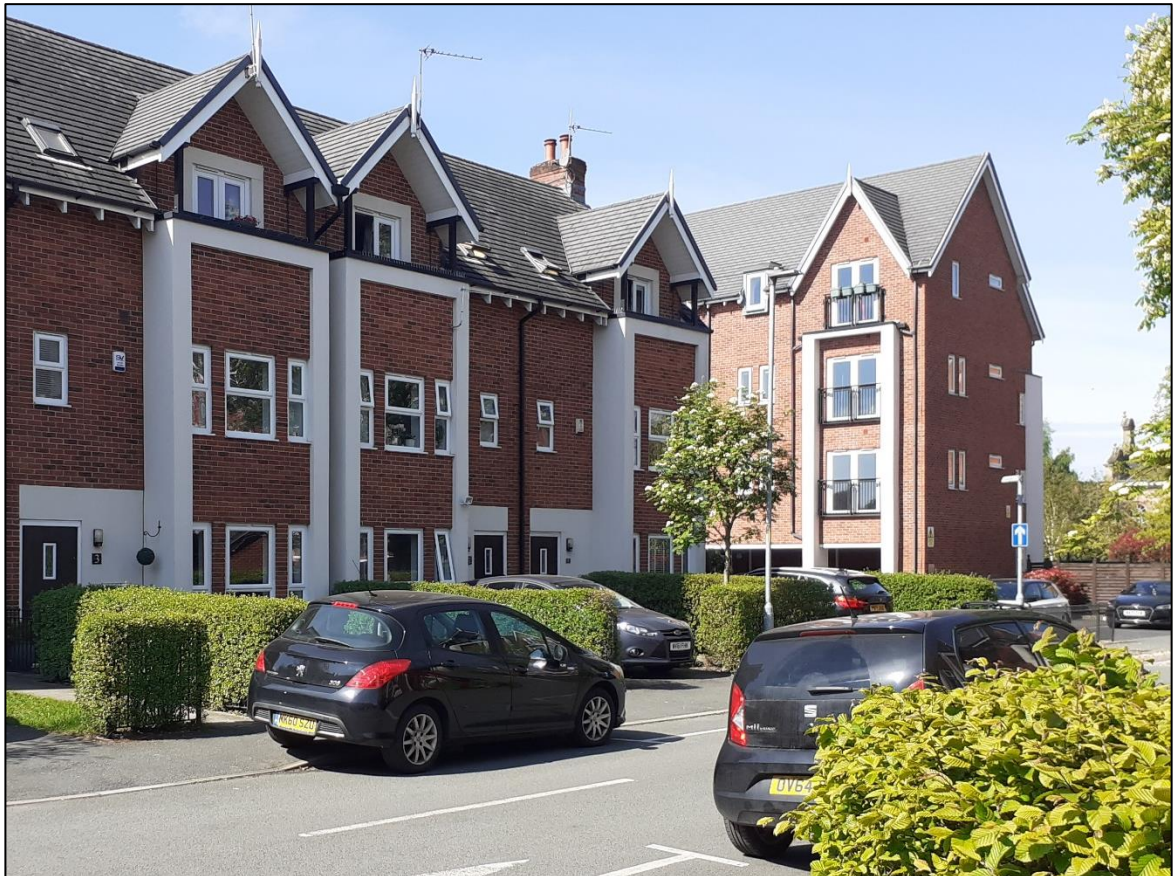
Figure 1: View of front elevation of the terrace block with 7 Hightrees Drive located at the end of the block. Four storey apartment development is visible in the background.
