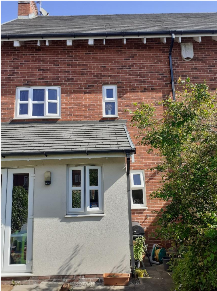
View of rear of 7 Hightrees Drive.
