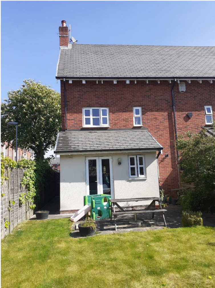
View of rear of 7 Hightrees Drive.
