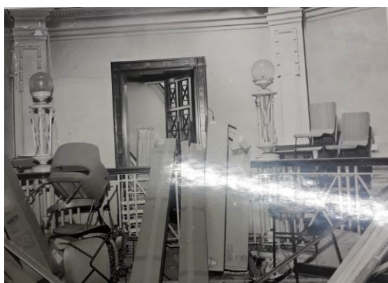
Gallery balustrading detail during the installation of the staff room floor, c1984.
