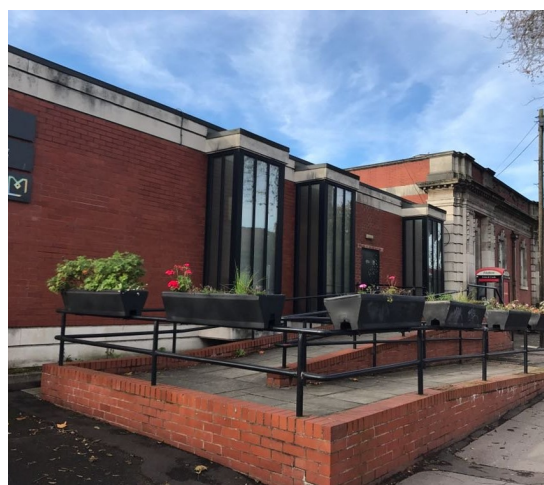
The east elevation of the 1964 extension to the Library building.
