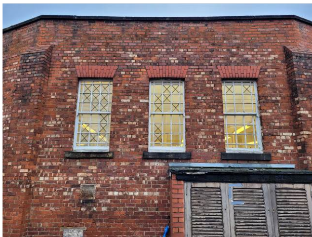
Plain detailing, rear elevation of the listed building.
