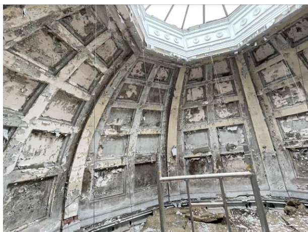
The dome above the suspended ceiling.
