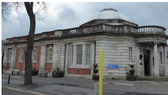
Portland stone and small gauge brickwork, east elevation.
