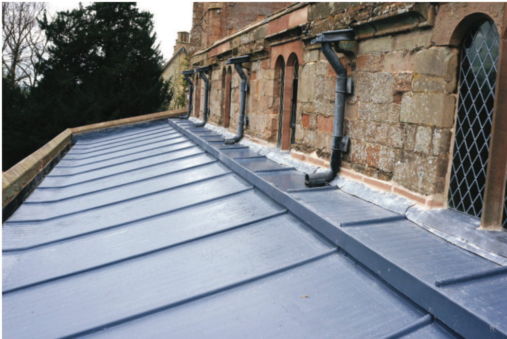
Use of GRP in a heritage setting as proposed
