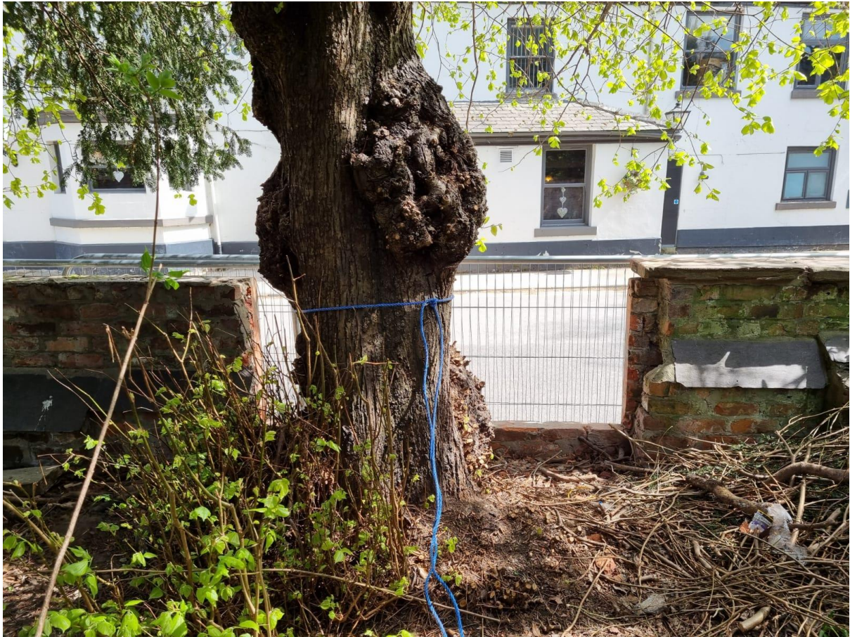
Photo 5: Section of boundary wall removed as part of the emergency works.
