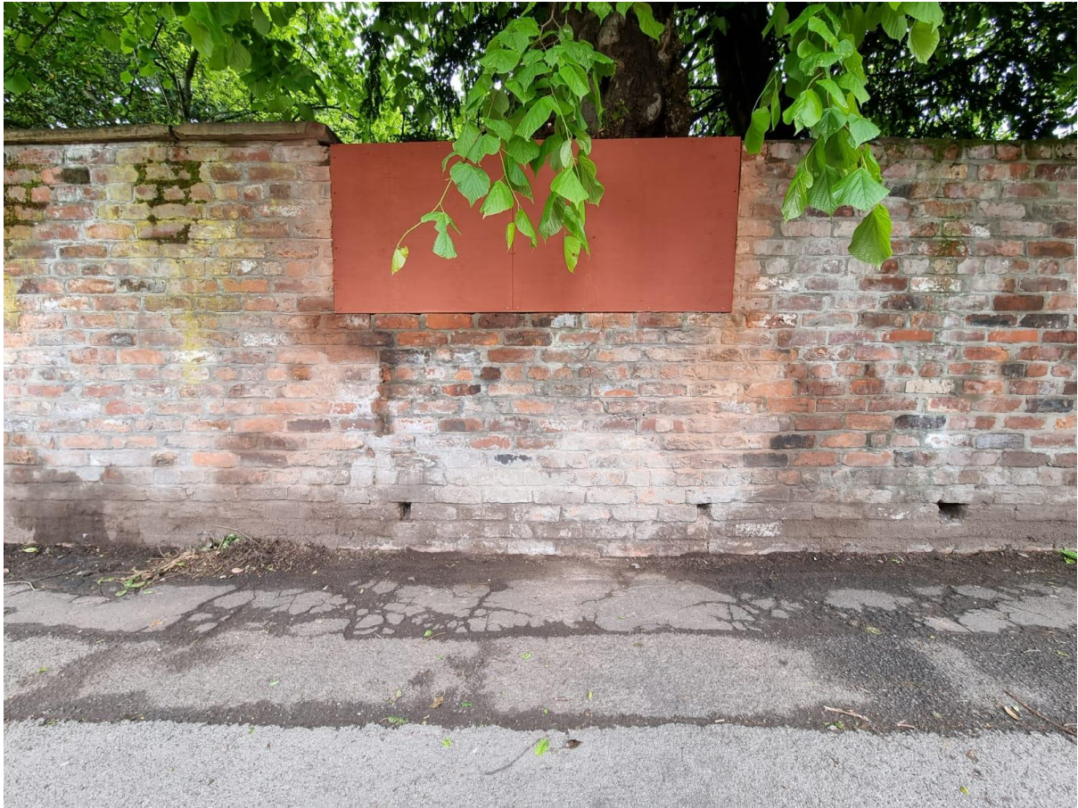
Photo 6: Boarded up section of wall put in place to temporarily secure the grounds.
