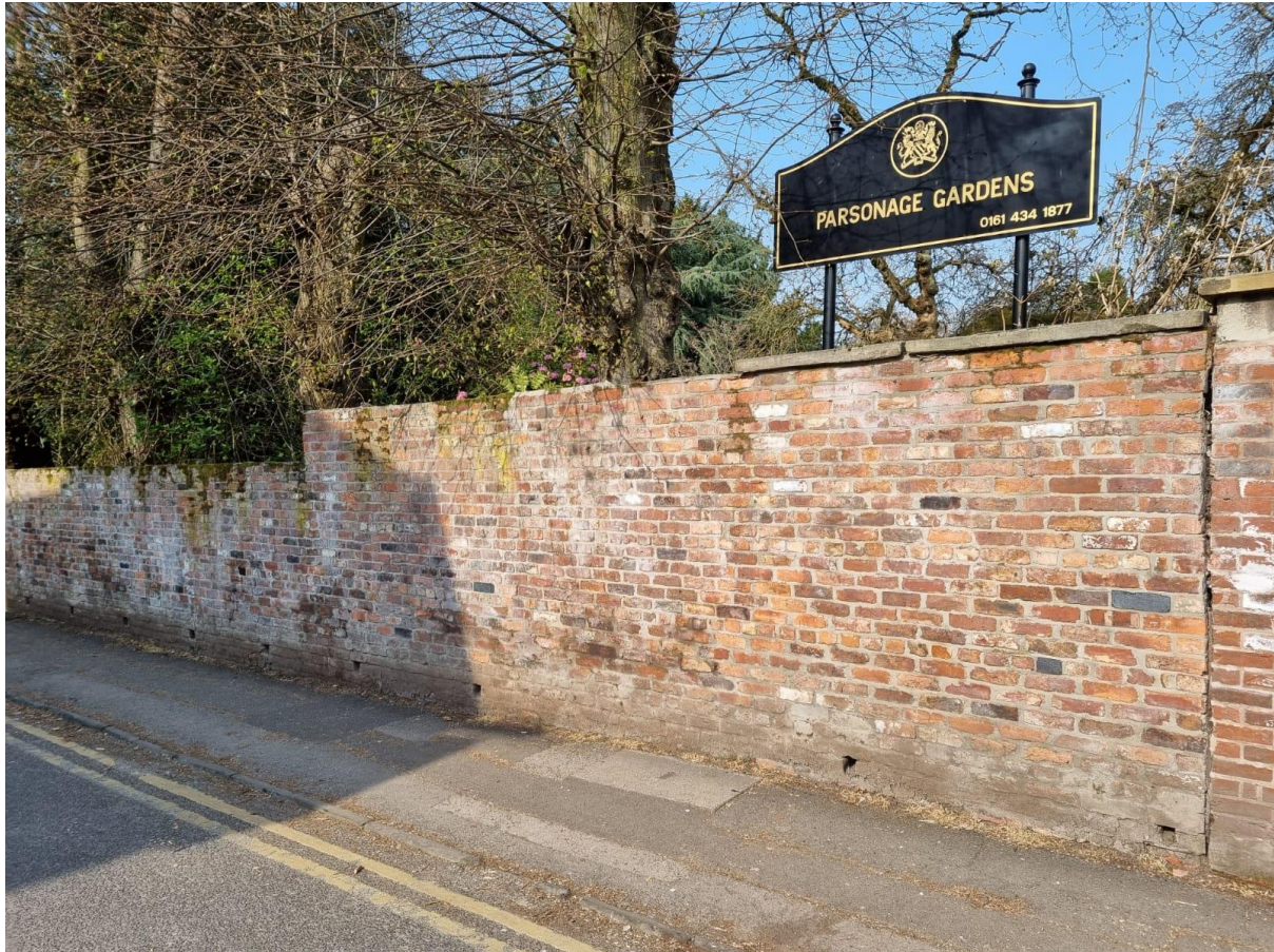
Photo 7: Existing section of wall to be dismantled and rebuilt to a reduced height to match attached lower section of boundary wall.
