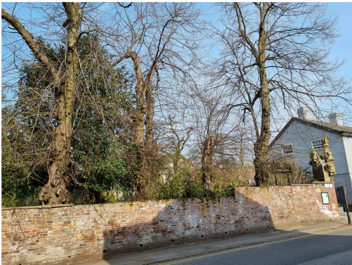
Photo 1: Photo taken on Stenner Lane facing the Eastern perimeter boundary retaining wall to Fletcher Moss Art Gallery.
