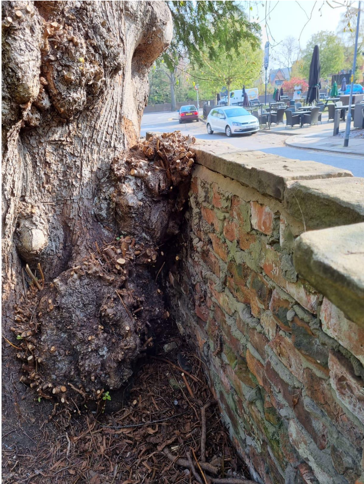
Photo 3: Lime tree adjacent to the boundary wall. This section of wall was removed as part of the emergency works.
