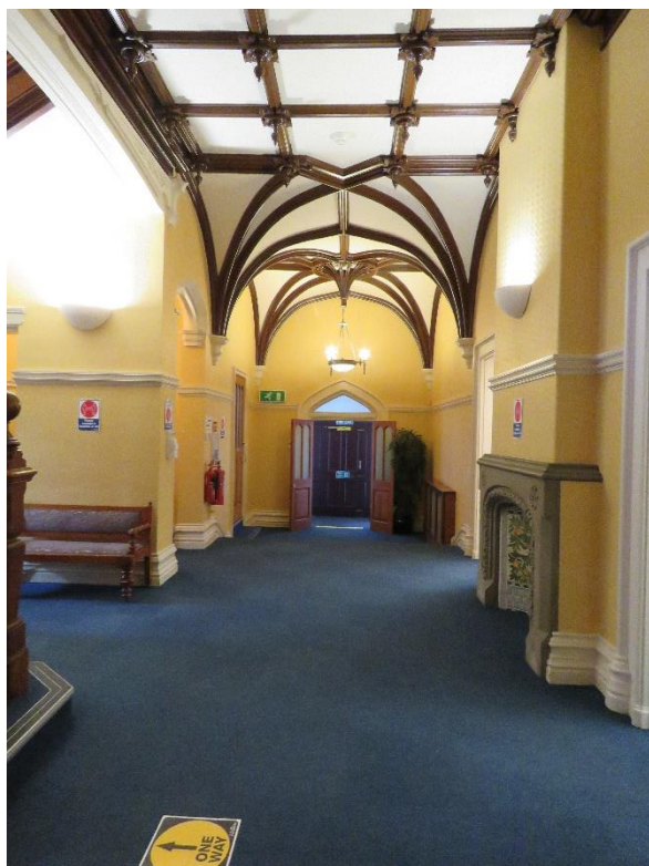
Figure T – Looking north towards the entrance porch from the stairs. Note the fireplace to the right and original high-quality joinery (skirtings, doorframes, ceiling etc)
