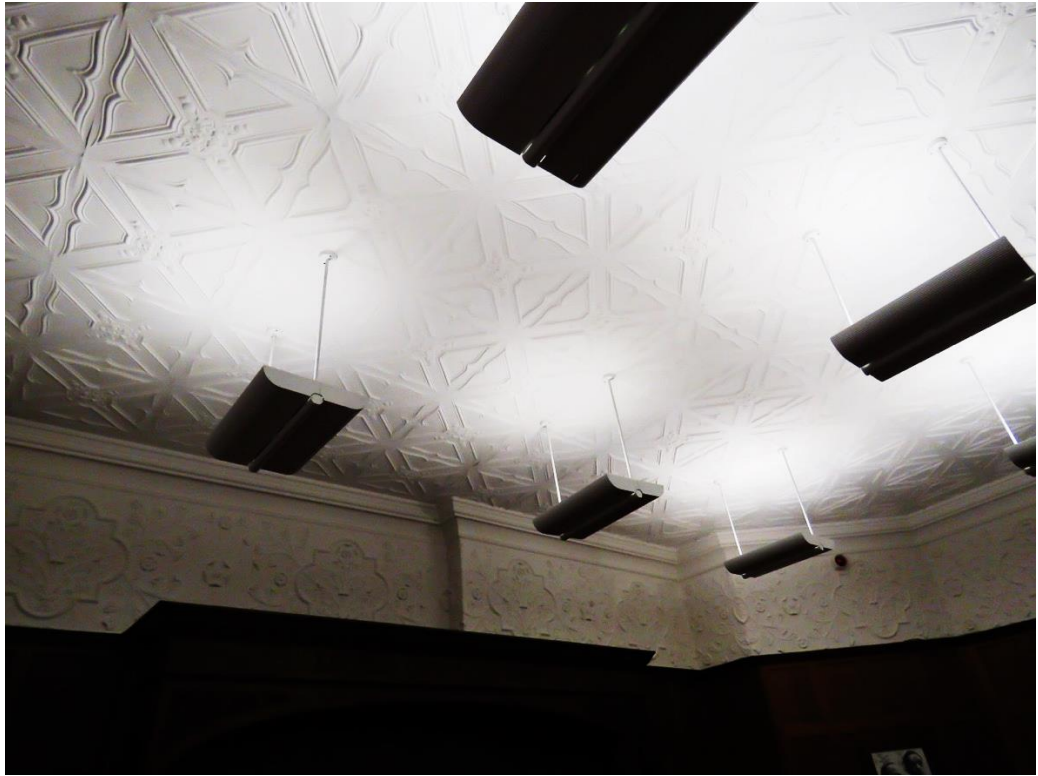
Figure DD – The decorative ceiling and frieze plasterwork.
