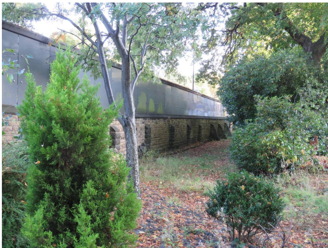
Figure Ni - The eastern boundary wall facing Wilmslow Road; note the modern bus shelter structure that screens the gardens and Appeal Site.
