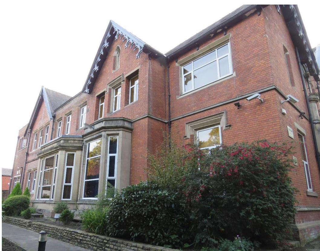
Figure M – The east elevation as seen in 2020 showing the subsequent removal of the original Gothic stone mullions to both ground floor bay windows.
