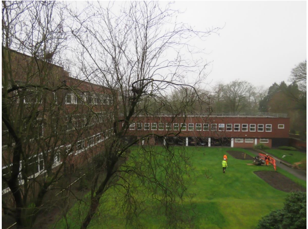
Figure F – The 1970s/80s extension to the west of the Site which cuts across the former gardens of the house.
