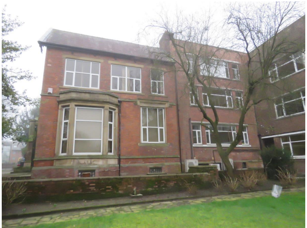
Figure C – The west elevation. Note the insertion of uPVC windows which detracts from the appearance of the house and the 1930s extension to the right which dominates the historic building.
