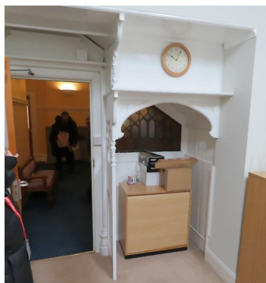
Figure X – The inside face of the internal window, which appears to have been inserted in the c1880s.
