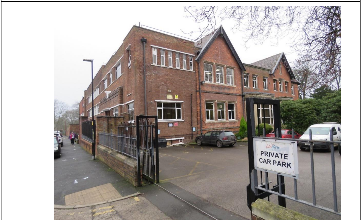
Figure B – The east elevation of Oakley (right) showing the 1937 extension to the left. Note
