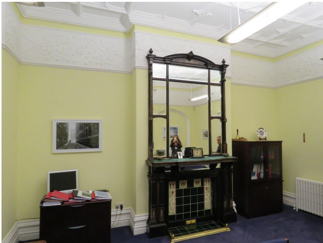
Figure EE – An original polished slate fire surround and over-mantle mirror to the east elevation of the ground floor, showing original c1837 Gothic ceiling plasterwork, and c1887 plaster frieze.
