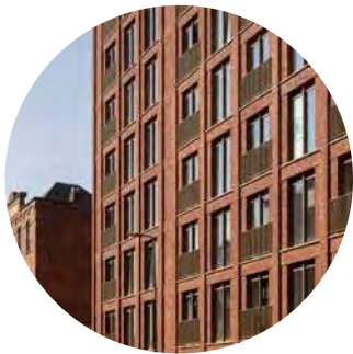
Brick deep window reveals add variation and depth across the facade
