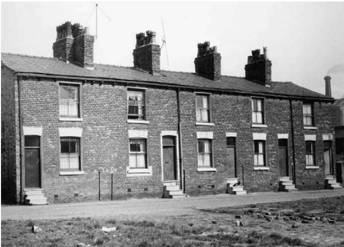
Ancoats, Kemp Street, Facing West (1962) - Manchester Local Image Collection
