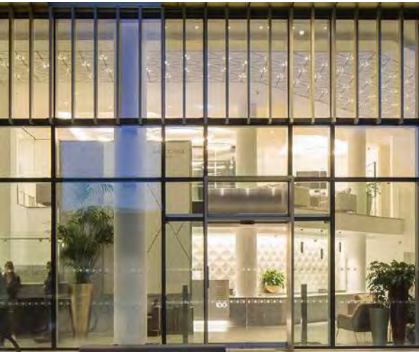
Curtain Walling to Ground Floor Entrances and Residents Amenity Spaces
