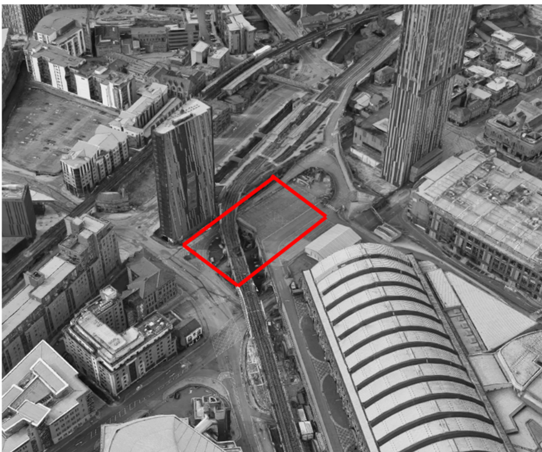
3D View of the site and the surrounding area
