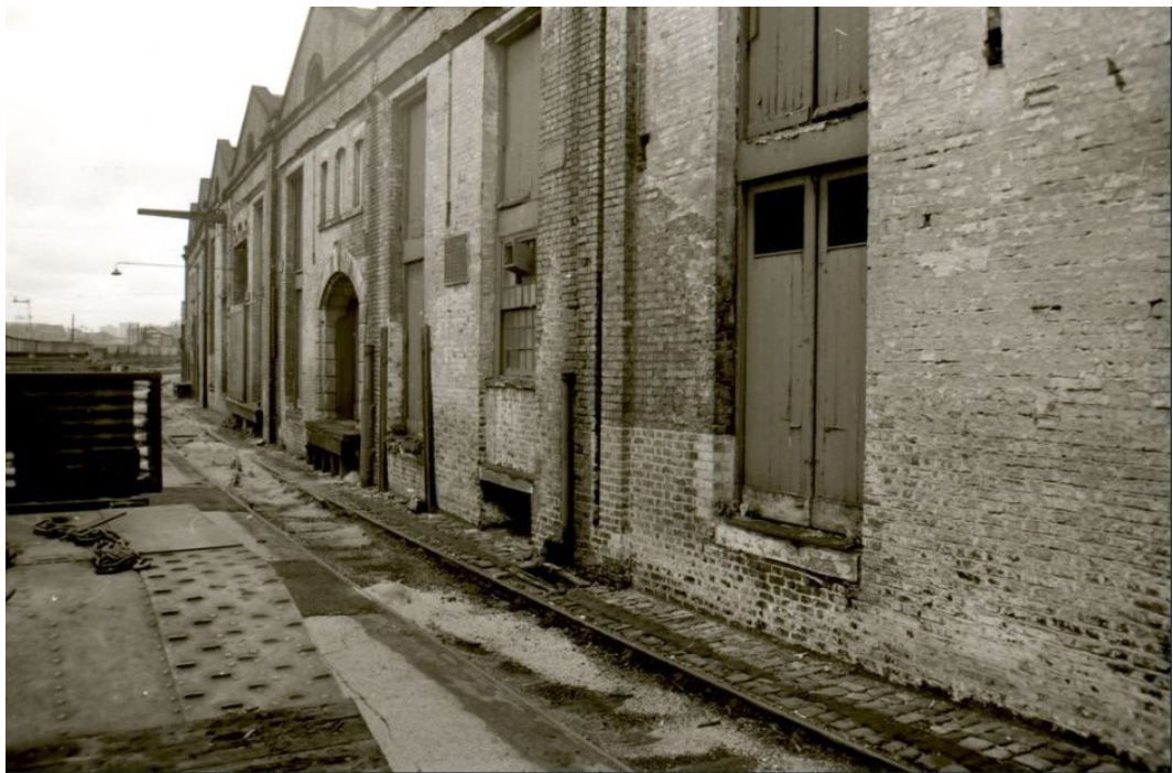
Figure 6: n.d photograph of the western part of the southern elevation (Manchester libraries, supplied by museum)
