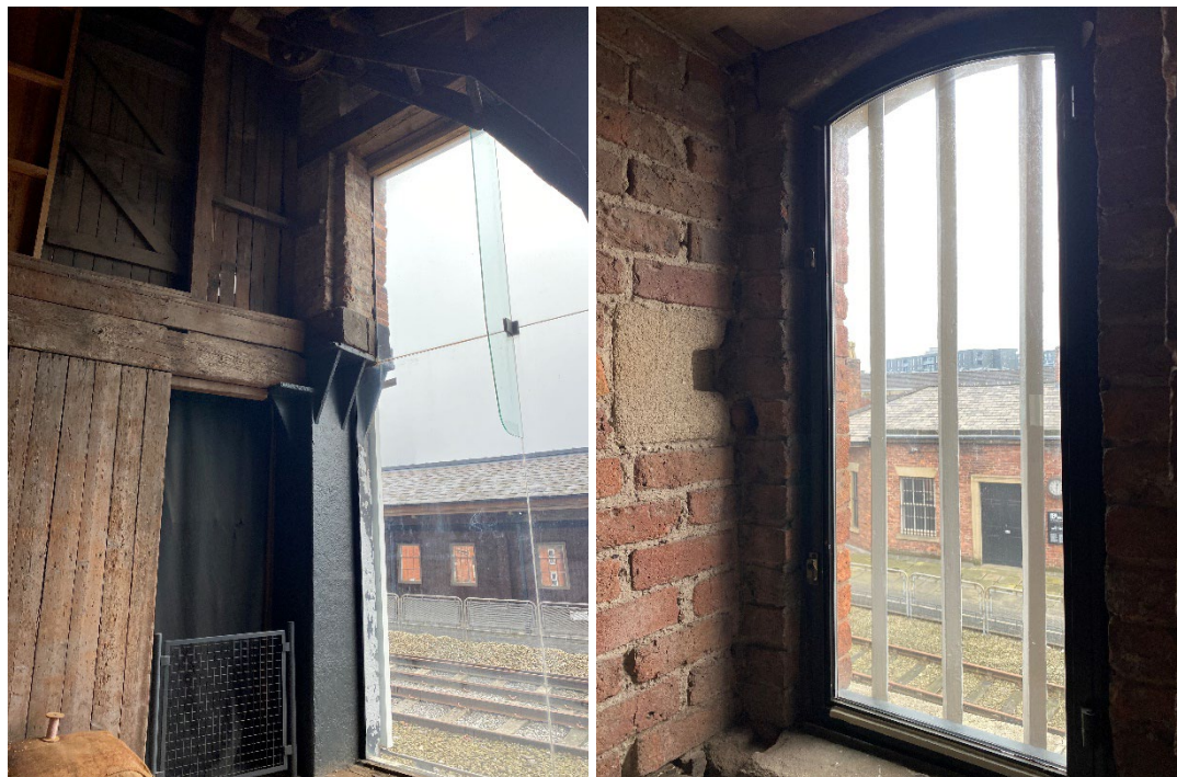
Figure 8-9: (left) frameless system installed within Bay 2; (right) example of typical framed windows inserted within the smaller windows in Bays 1-3.
