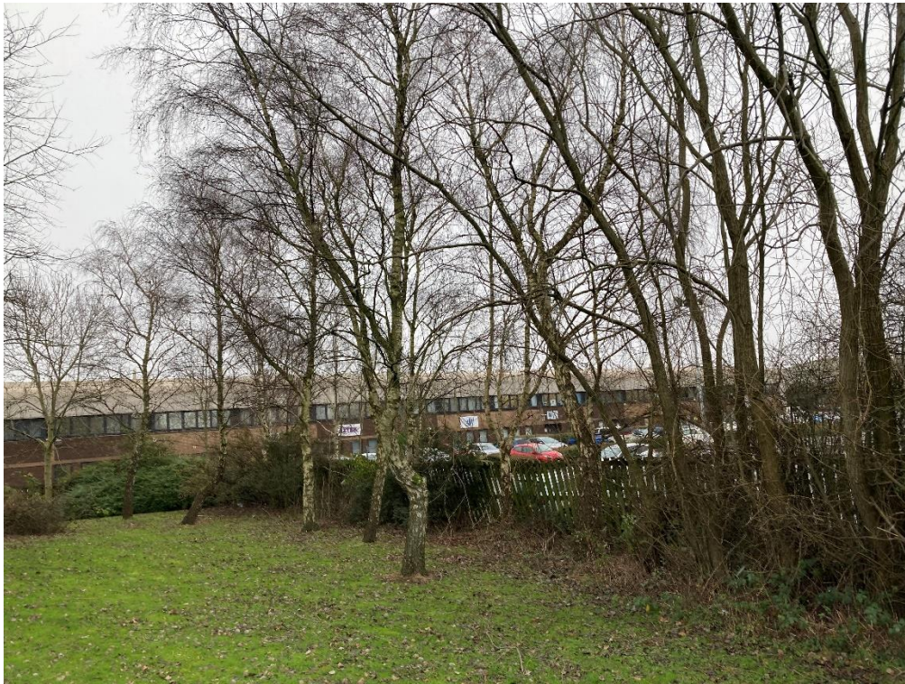
Image 4 South east view of G5 with G4 on the left in the background
