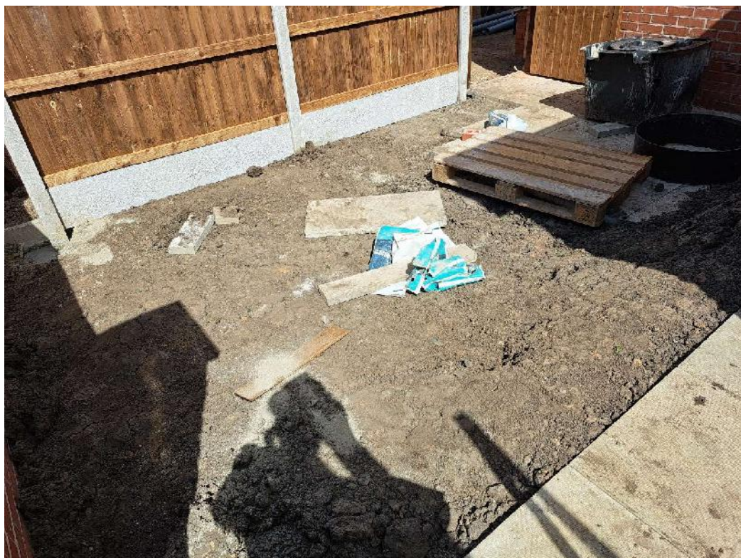
Photograph 16 Overview of rear garden of Plot 10.
