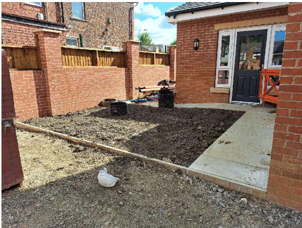
Photograph 14 Overview of rear garden of Plot 04.
