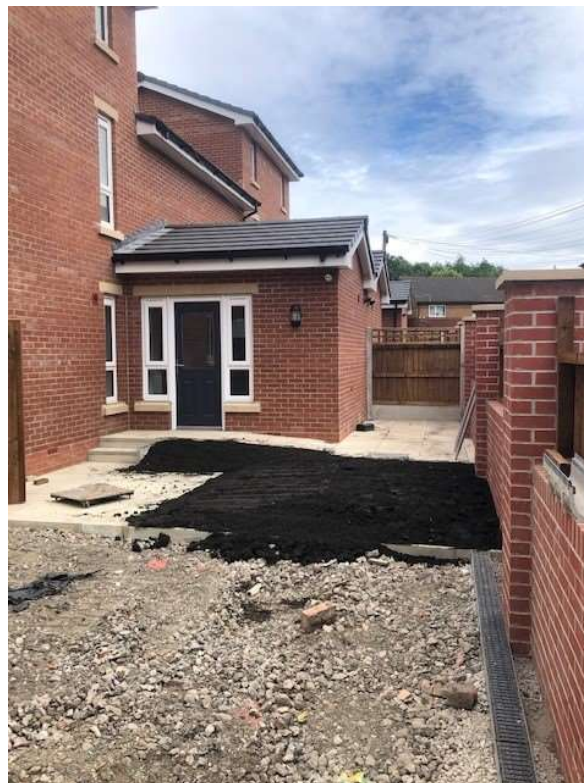
Photograph 18 Overview of rear garden of Plot 08 taken 12/07/22.
