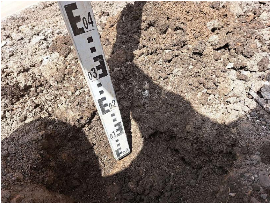
Photograph 7 250mm of topsoil emplaced in VP03.
