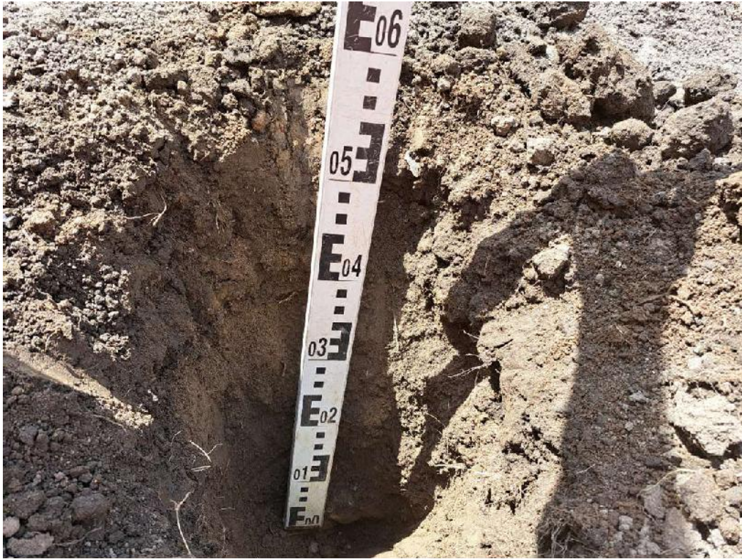
Photograph 5 350mm of subsoil emplaced in VP02.
