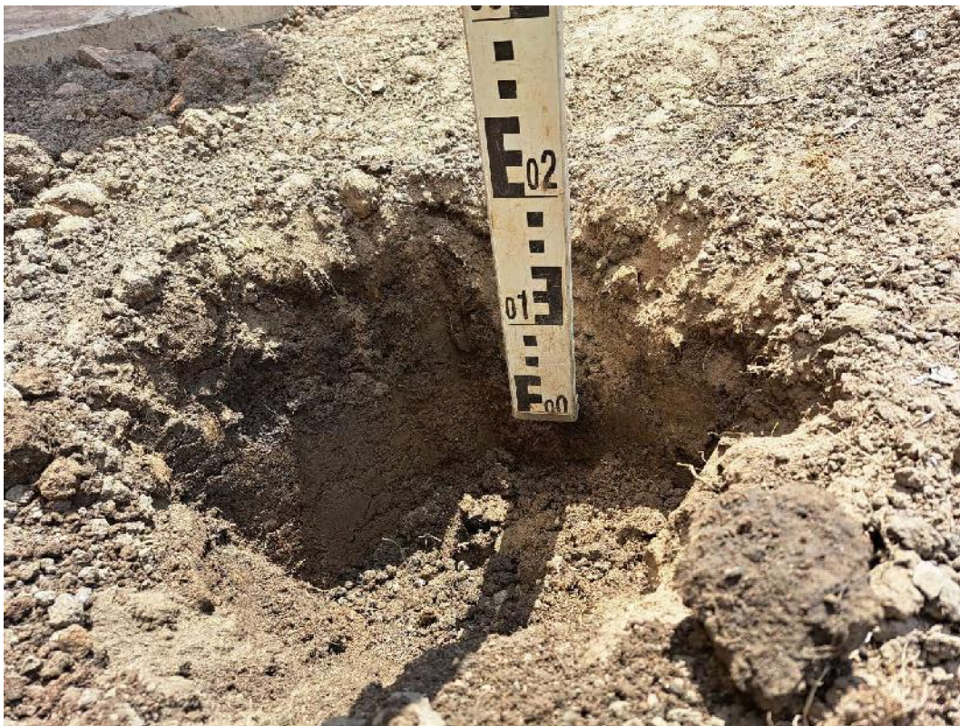
Photograph 10 200mm of topsoil emplaced in VP04.
