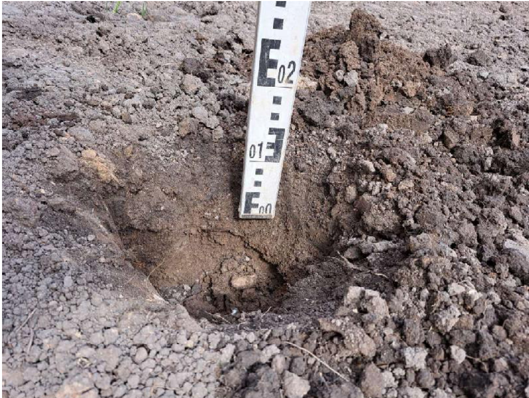
Photograph 1 150mm of topsoil emplaced in VP01.
