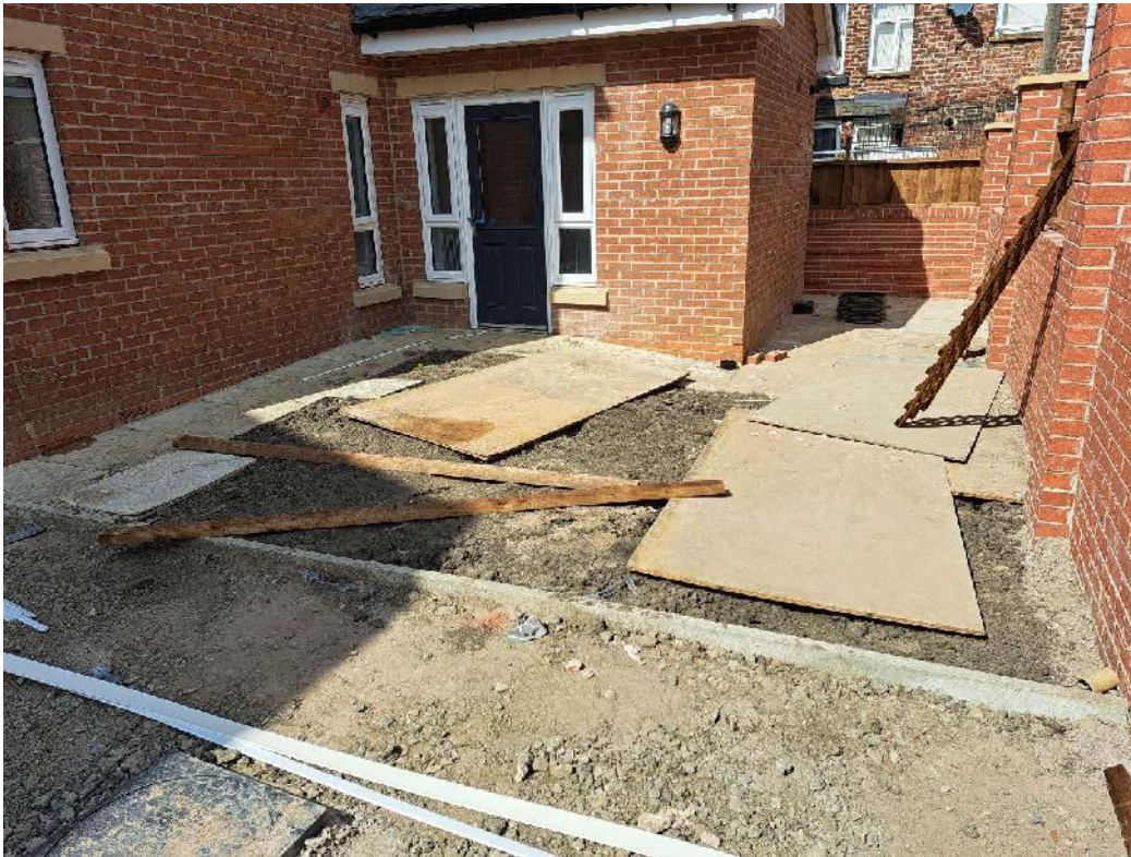
Photograph 13 Overview of rear garden of Plot 01.
