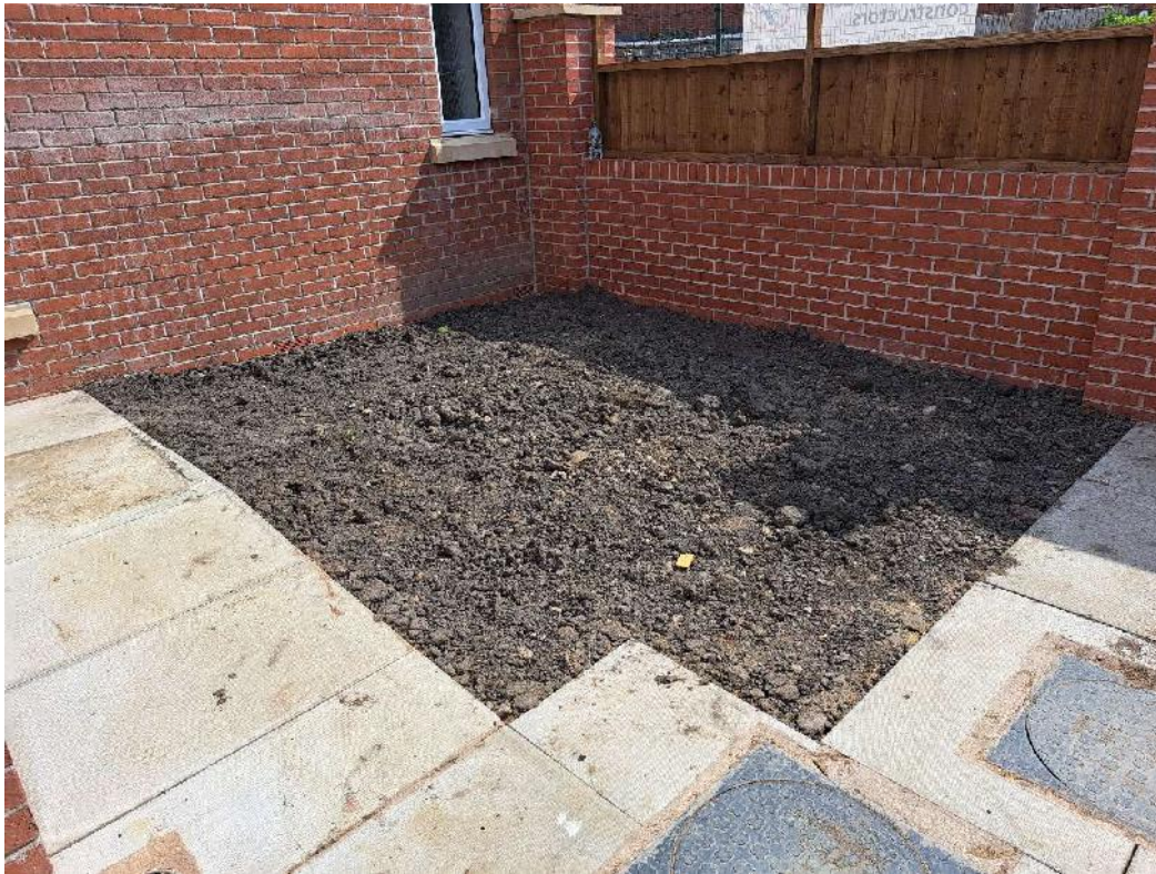
Photograph 15 Overview of rear garden of Plot 06.
