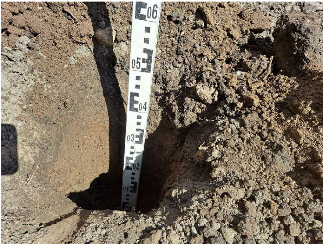
Photograph 2 400mm of subsoil emplaced in VP01.
