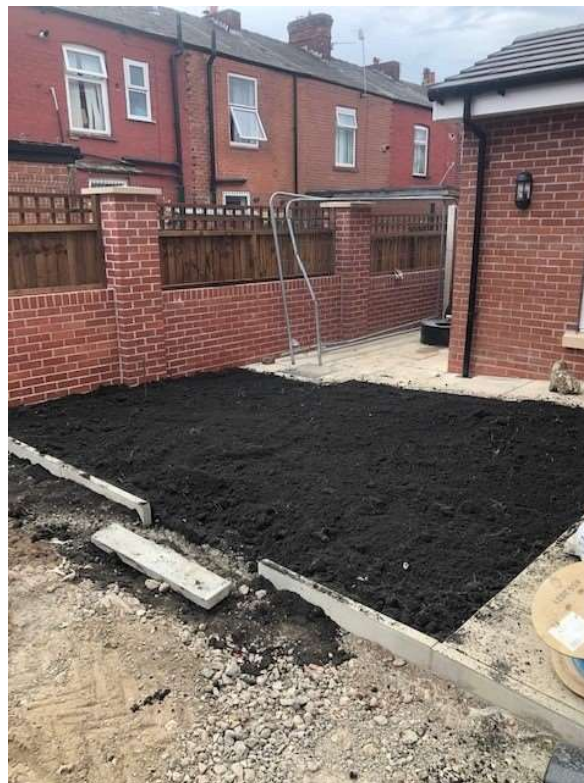
Photograph 20 Overview of rear garden of Plot 09 taken 12/07/22.
