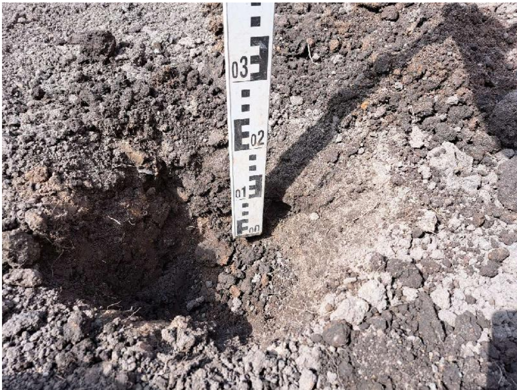
Photograph 4 200mm of topsoil emplaced in VP02.
