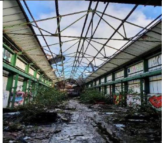
Photograph 6: Internal of B1
