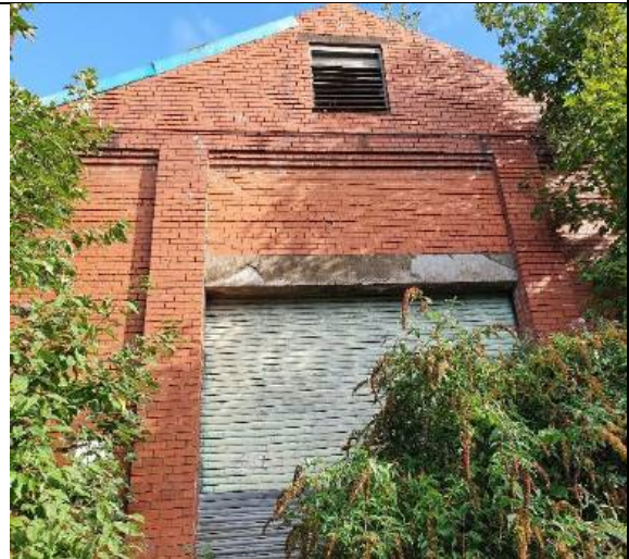
Photograph 4: Southern elevation of B1
