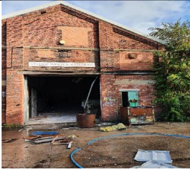
Photograph 7: Southern elevation of B2
