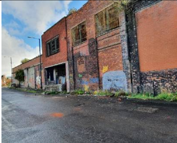
Photograph 5: Western elevation of B1
