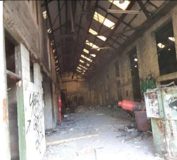
Photograph 8: Internal of B2
