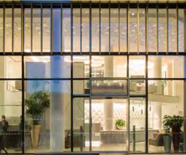
Curtain Walling to Ground Floor Entrances and Residents Amenity Spaces
