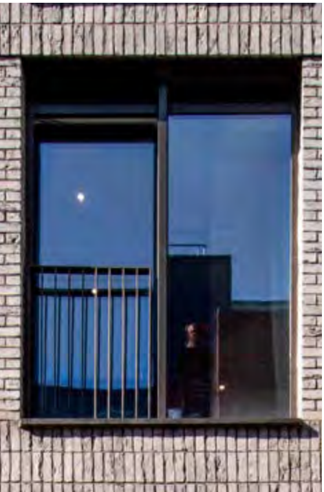
Aluminium grey window frames and juliet balconies
