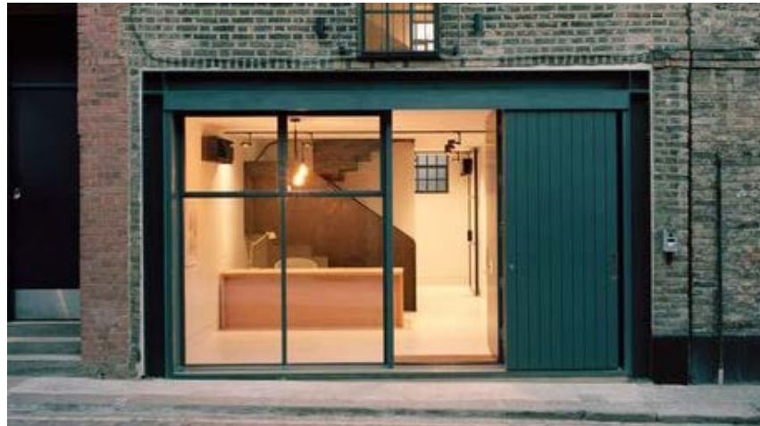
Retail shopfront recessed from brick facade
