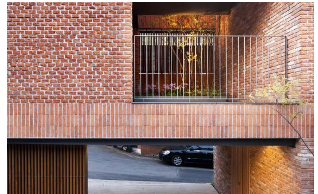
Feature brick detail above shopfronts
