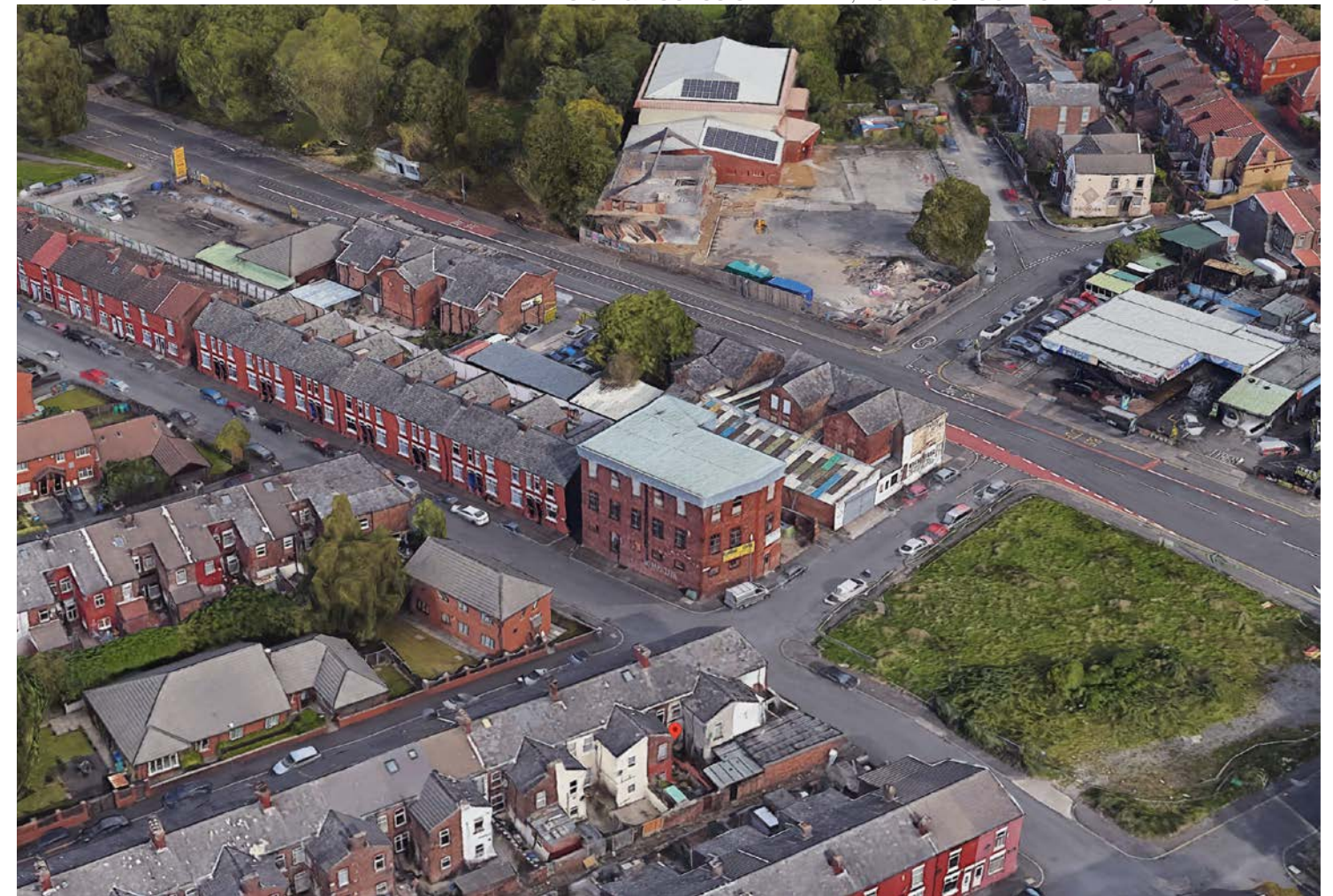
Aerial view of site, corner of Siddall street and Swallow street
