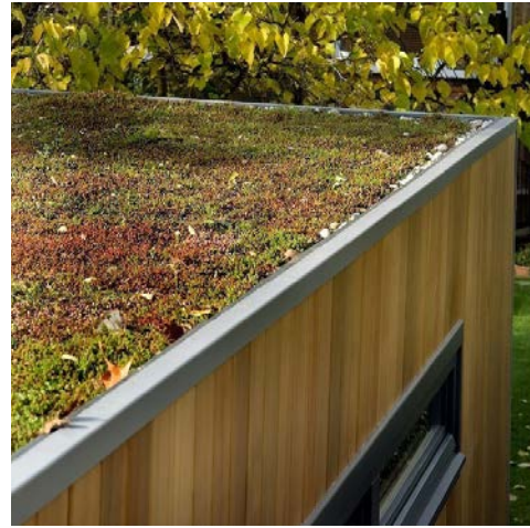
Modular sedum green roof
