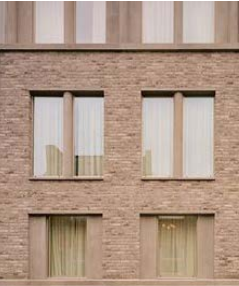
Double windows with precast mullions
