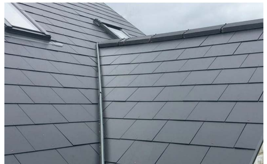
Fibre Cement Roof Tiles to houses
