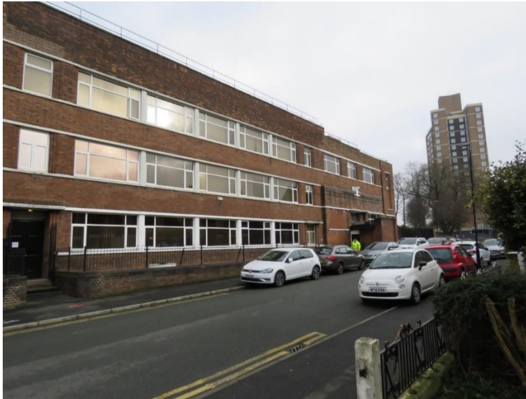
Photograph of existing ribbon windows that overlook existing terrace houses
