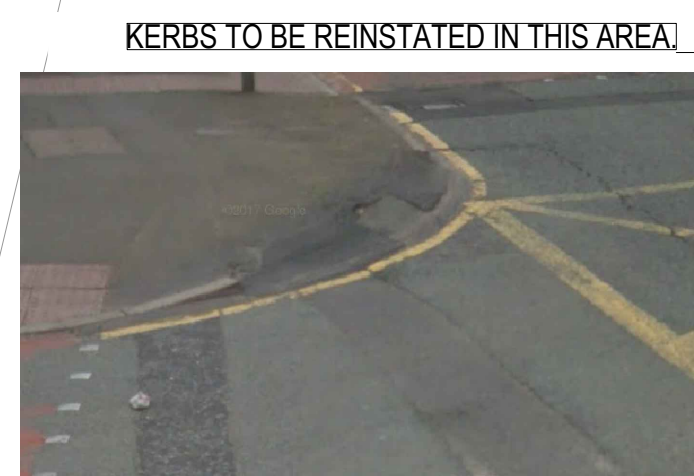
KERBS TO BE REINSTATED IN THIS AREA
