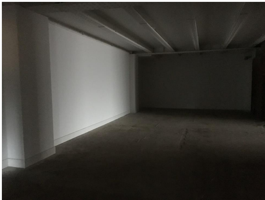
Figure 8: Example of Original Columns to Level 2 (overcovered in plasterboard c.2017 – July 2018). Pictured here in March 2019.
