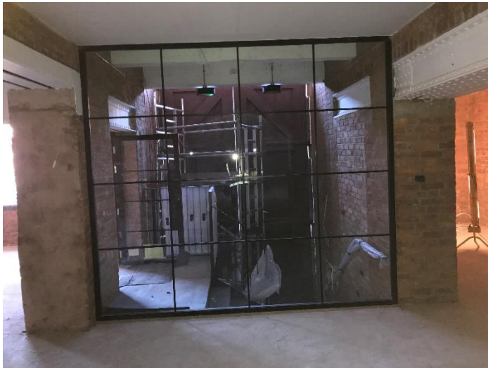
Figure 9: example of modern glazed partition installed c.2017 – July 2018 following Allied London's acquisition of the site.
