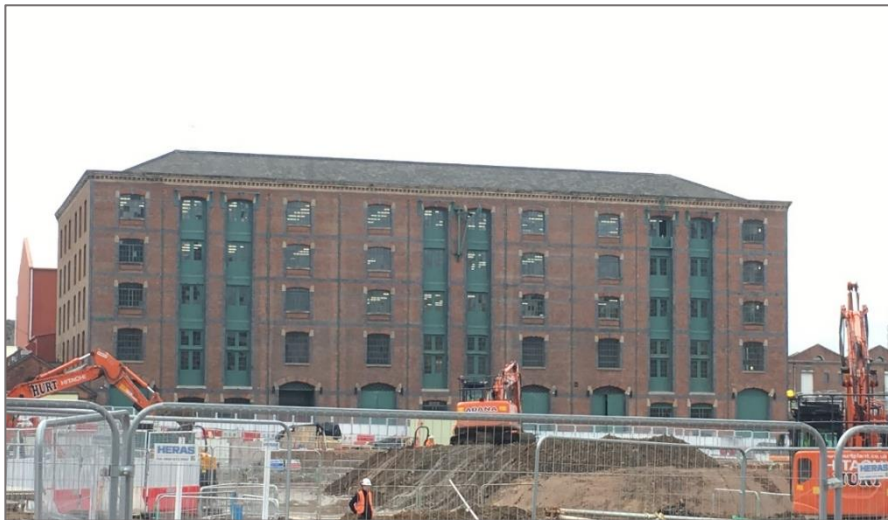
Figure 1: The Bonded Warehouse, north elevation, as seen in an oblique view from March 2019. (SLHA).
