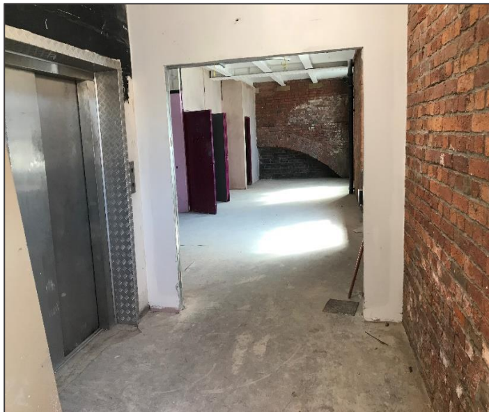
Figure 6b (top left): Example of modern lift core of no heritage significance. Installed by Granada Studios c.late 20 th / early 21 st century. Pictured here in 2017.
