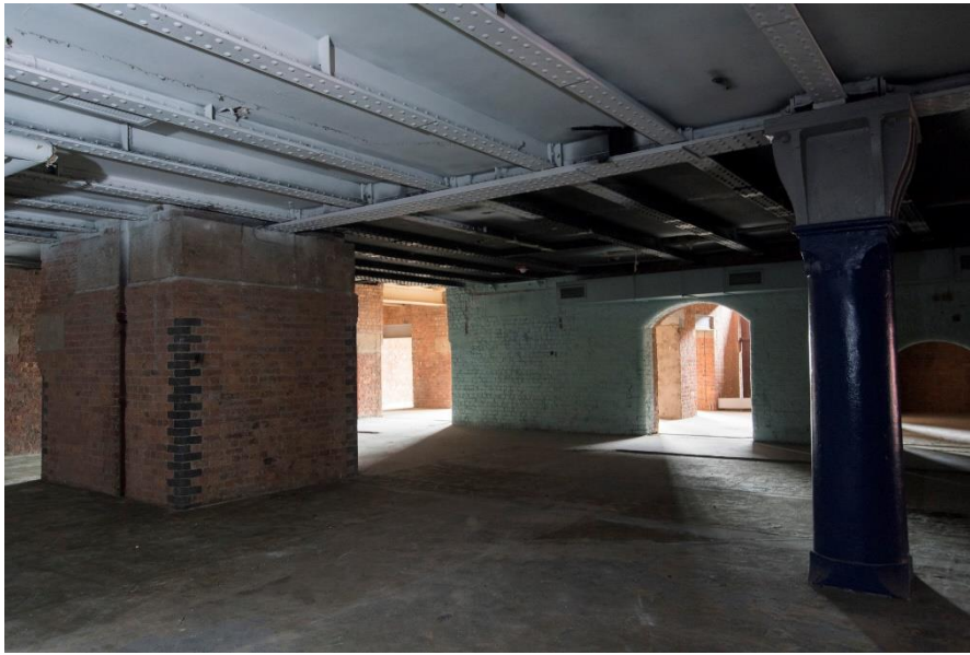
Figure 2: Level 2 of the Grade II Listed Bonded Warehouse. Pictured in 2017. Image provided by OBI.
