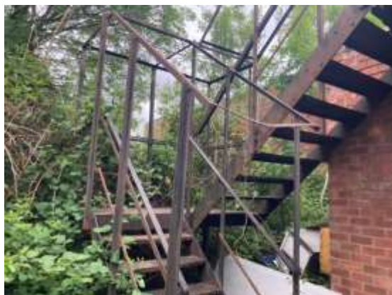
Partial rear view
