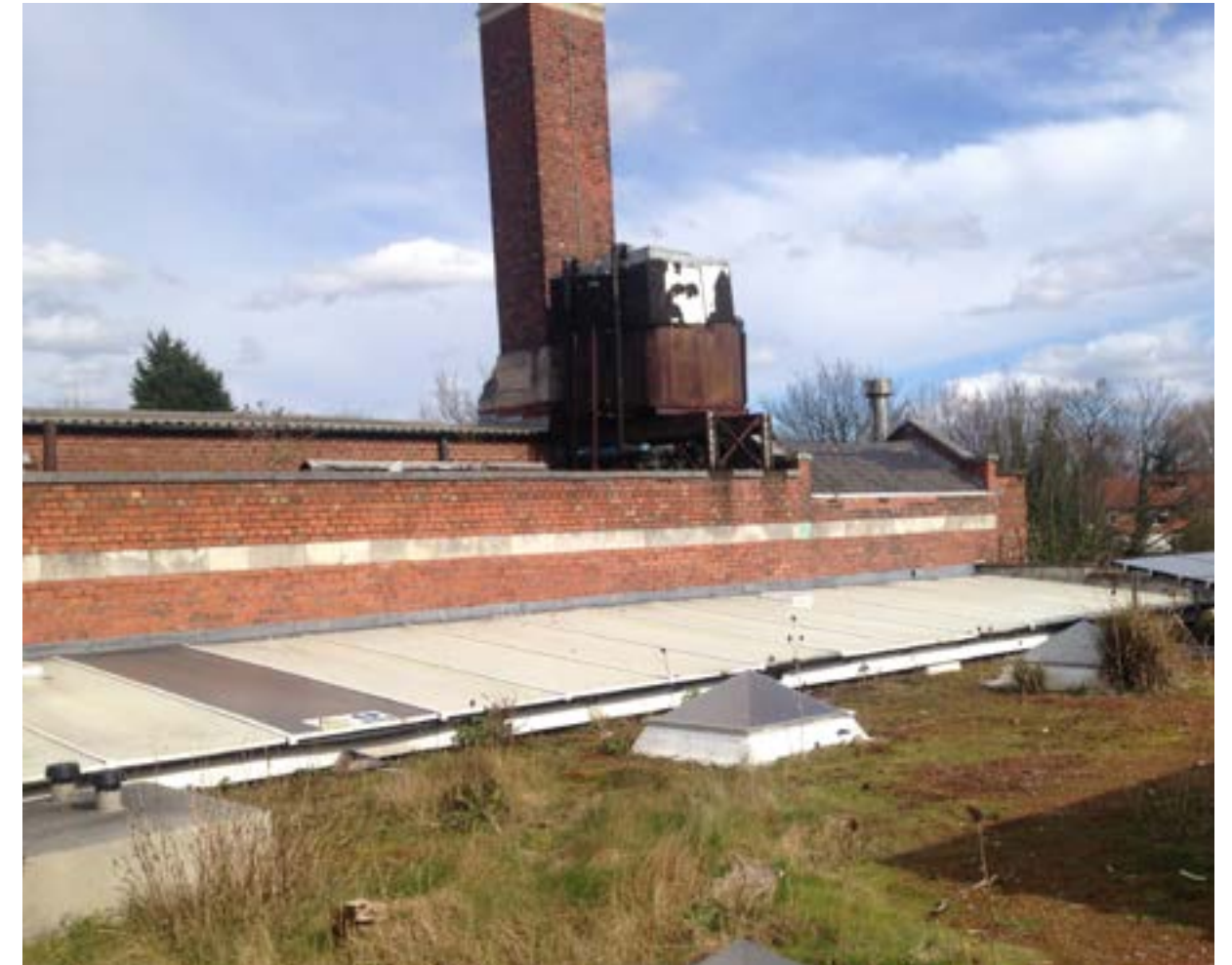
View of roof of existing lean-to from green roof, with existing baths wall in the distance.
