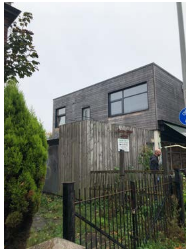
Existing fence to Manchester Road and earlier first floor extension with timber cladding.
