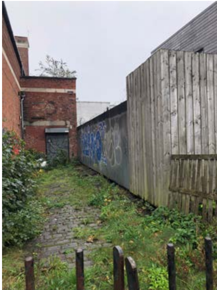
Existing fence to Chorlton Baths site from Manchester Road, white-painted brick parapet to existing lean-to.
