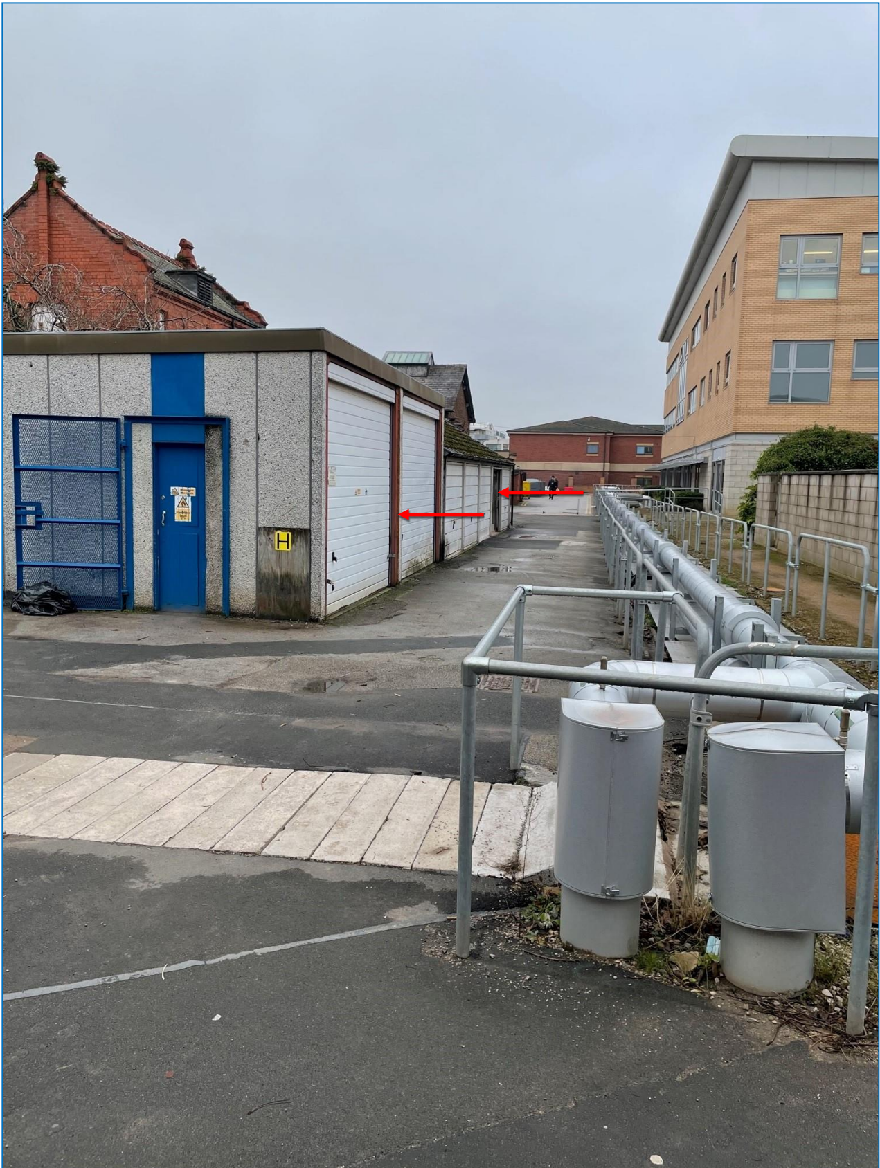
Fig. 4 Showing single storey buildings to be demolished prior to the commencement of the chimney demolition
