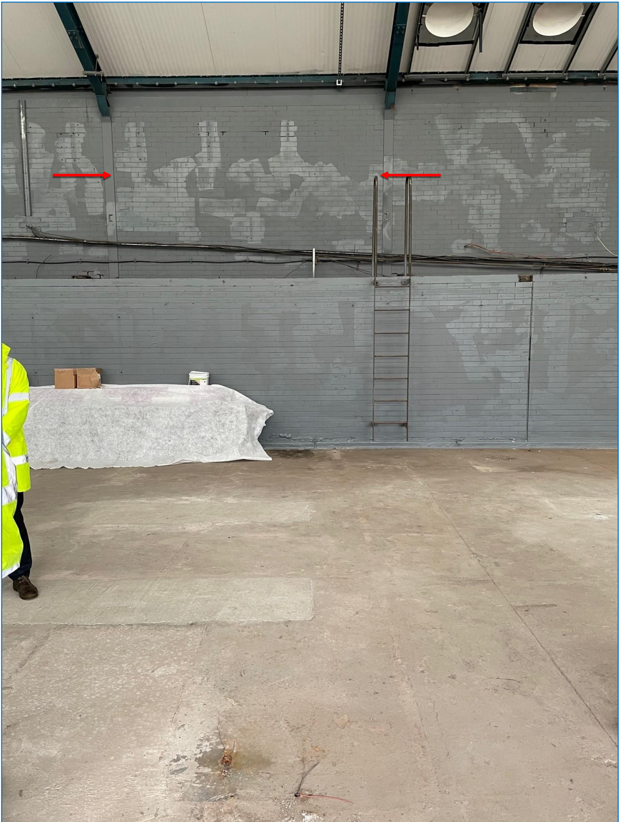
Fig. 3 Showing boiler house wall which will need to be removed prior to the commencement of the chimney demolition
