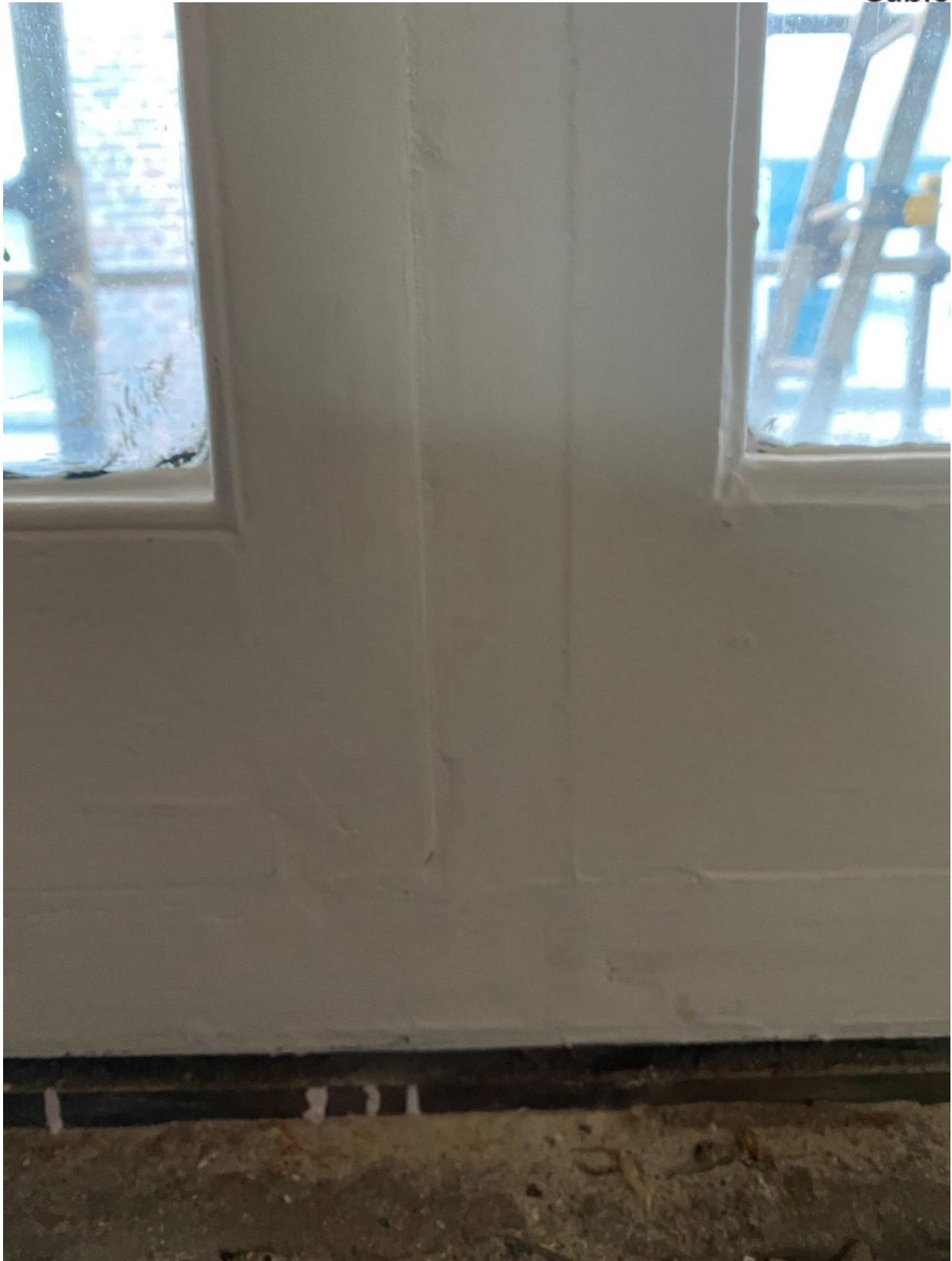
Figure 6 - Window painted after repairs (Credit CubicWorks Ltd.2022)
