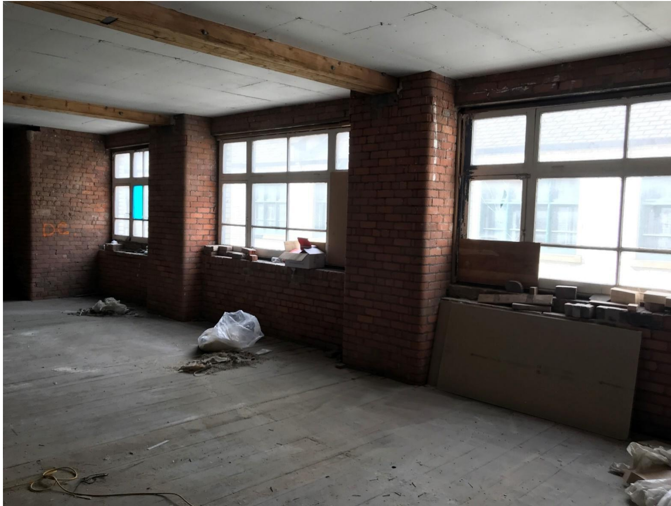
Figure 26: Brick Piers 2 (Credit CubicWorks Ltd.2022)
