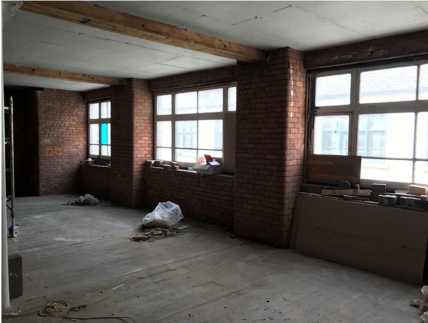
Figure 27: Brick Piers 3 (Credit CubicWorks Ltd.2022)
