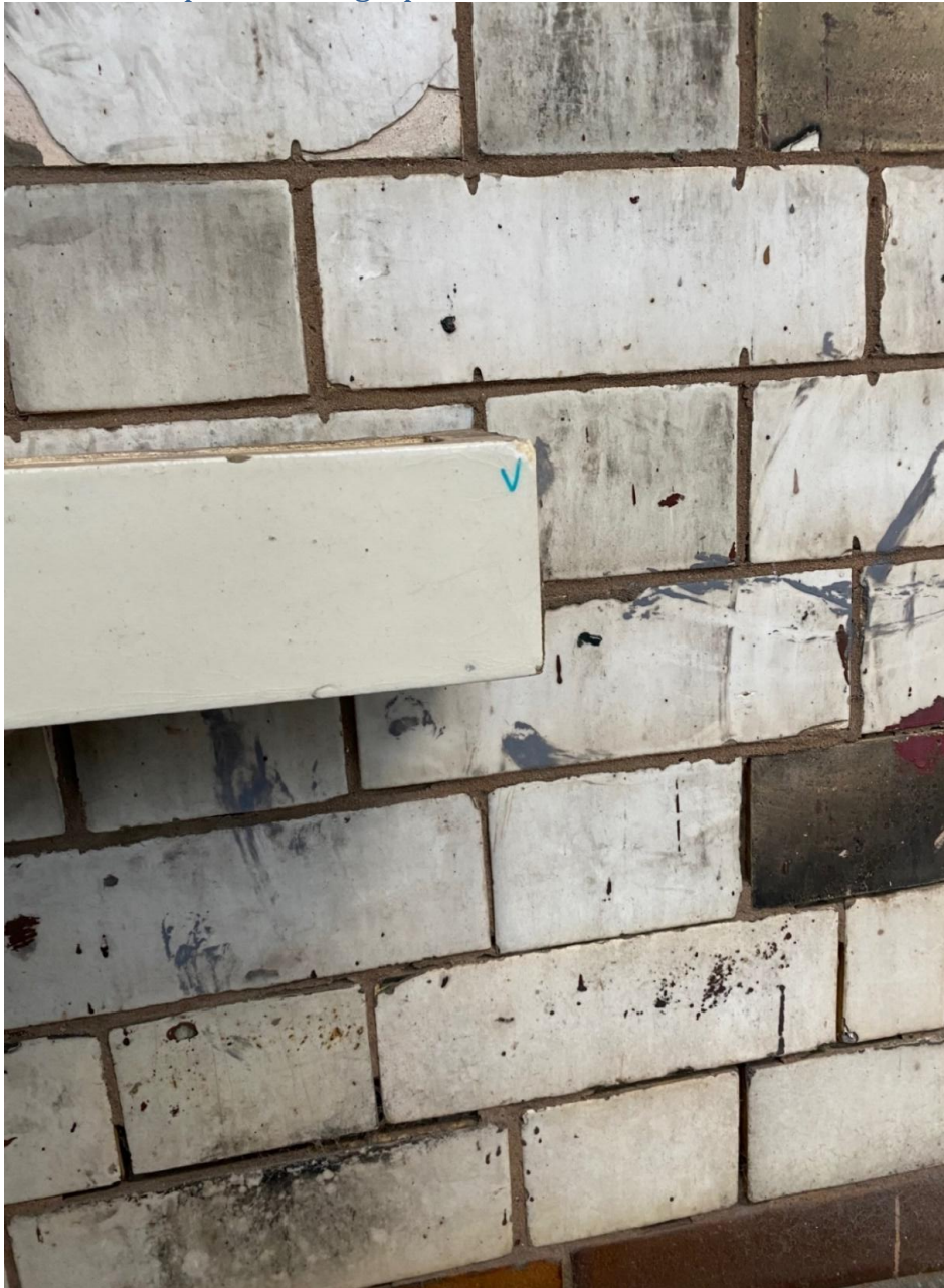
Figure 11: Parapet Wall rebuild ( Credit CubicWorks Ltd.2022)
