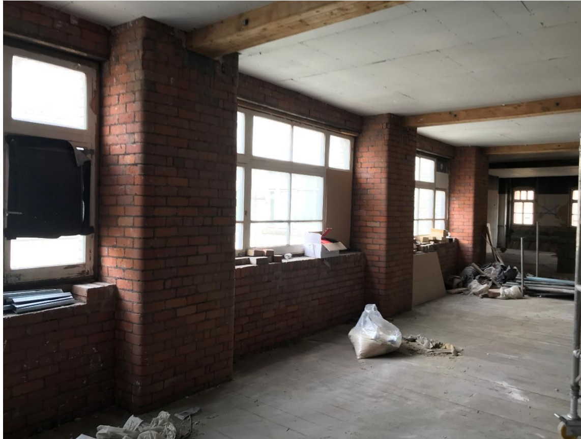
Figure 25: Brick Piers 1 (Credit CubicWorks Ltd. 2022)
