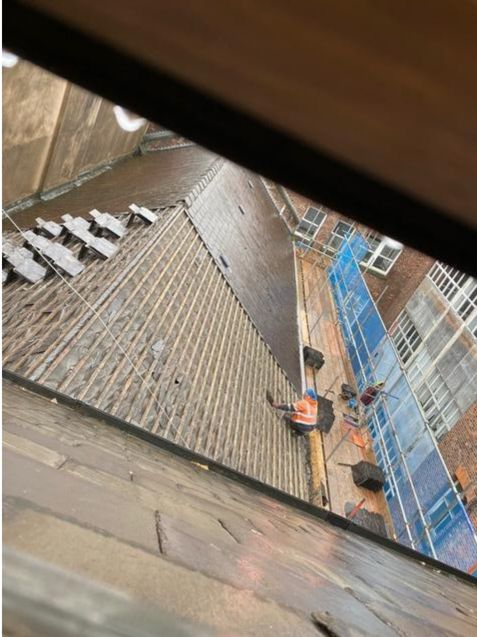
Figure 14: Slate removed from the original Mansard roof to be reused (Credit CubicWorks Ltd. 2022)
