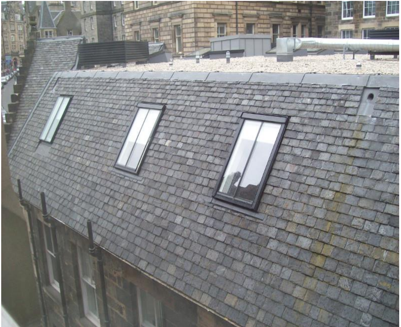
Figure 15: Fakro Conservation Roof Window example used in the multi-award winning Advocate's Close project in Edinburgh (Credit Fakro 2022)
