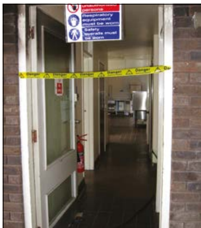
Make sure you restrict access
