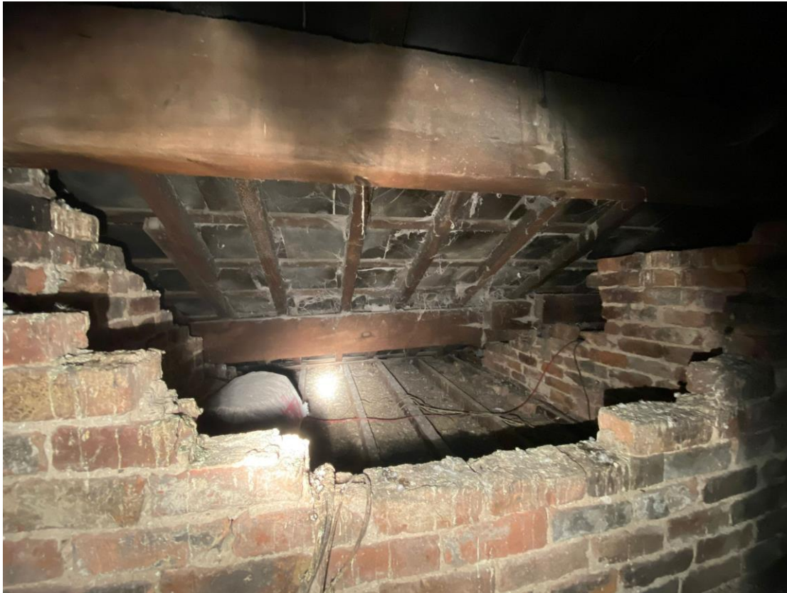
Photograph 13 – Open brick sectioned section located within section 1 of the loft void, with timber purlin rafters and bitumen lining.
