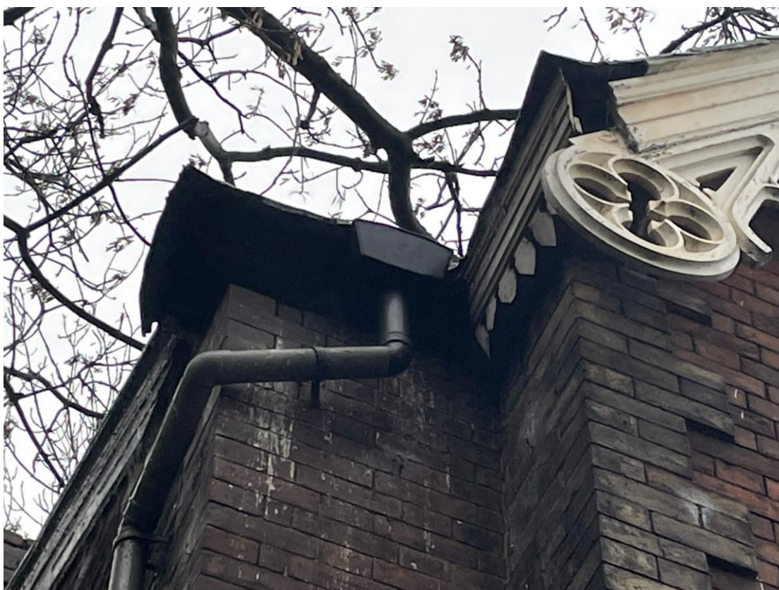
Photograph 4 – Northern aspect where access to the wall plate is granted by gaps in the fascia and barge board.
