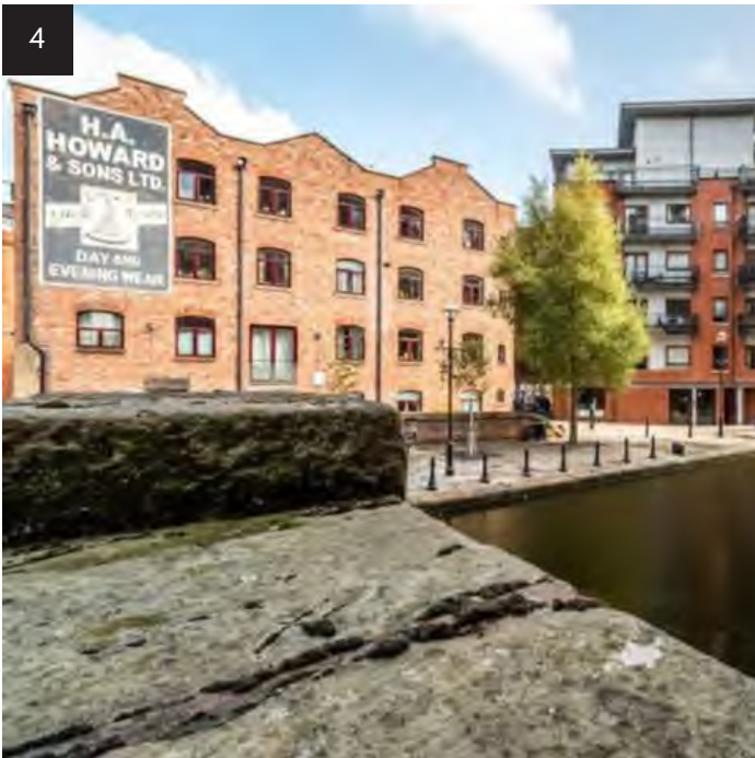
View from Ducie Street bridge towards Junction Works Apartments
