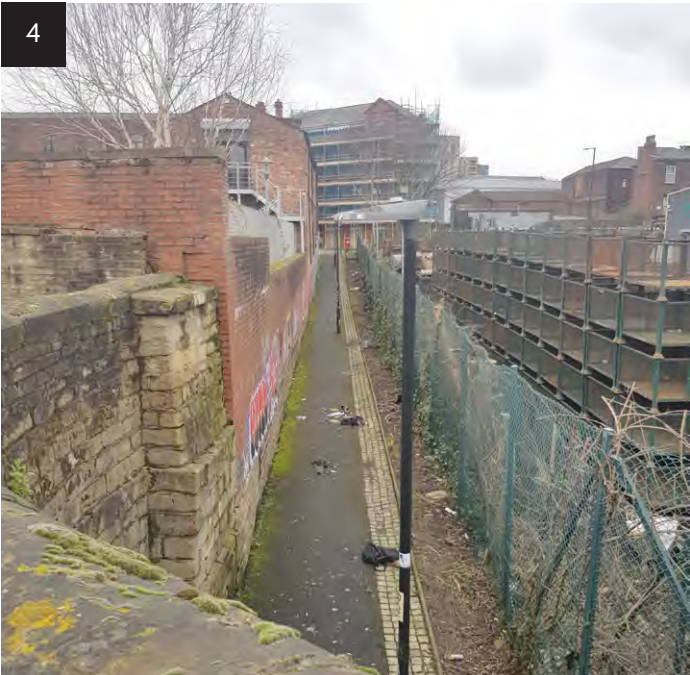
Northern view overlooking the condition of Paradise Walk
