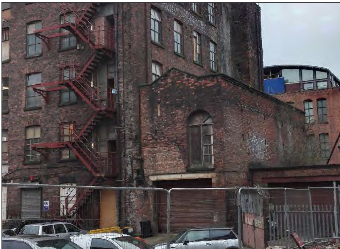
Plate 10: View of the engine house (Building 5), and modern structure on the site of the boiler house (Site 6)
