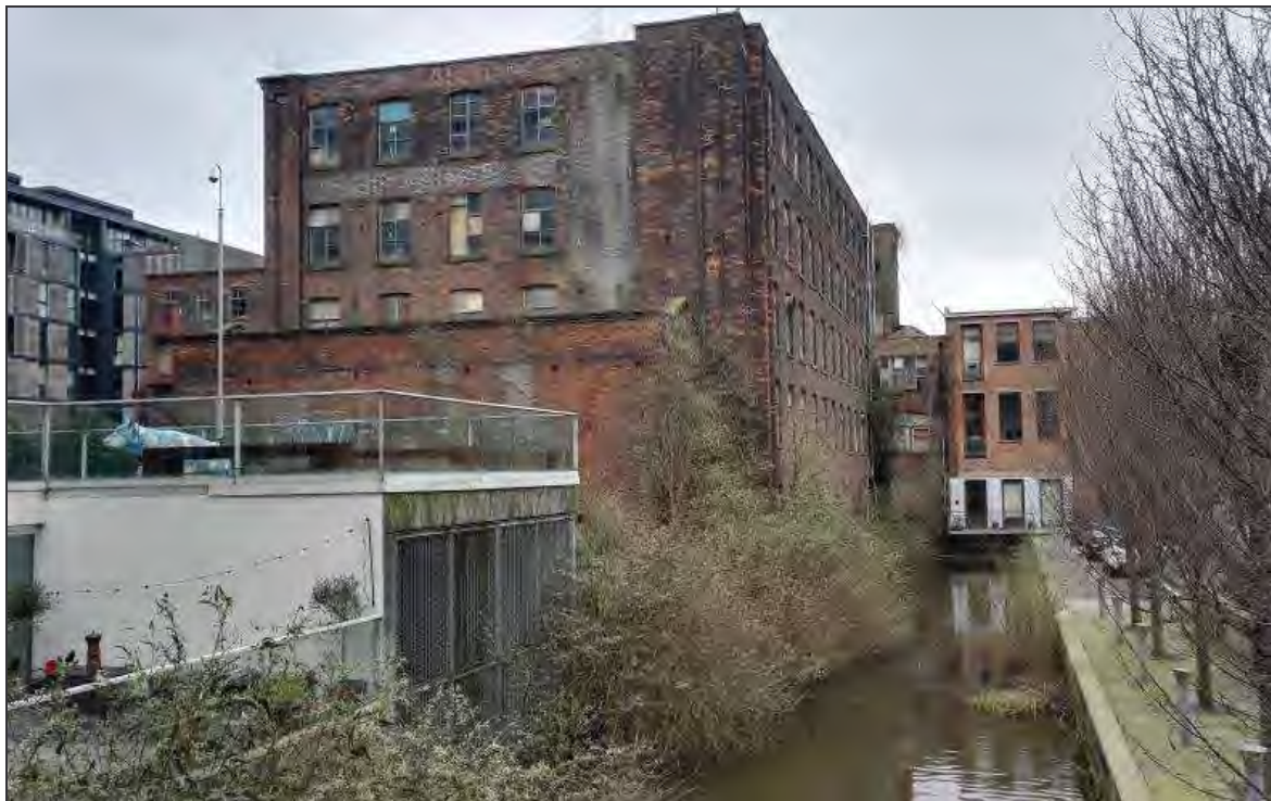
Plate 12: View of the canal arm that forms the western boundary of the Site Area
