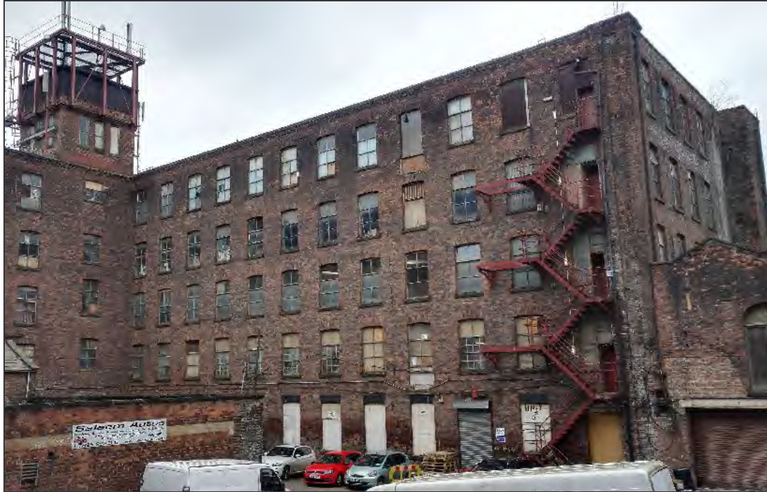
Plate 7: View of Mill 02 (Site 1) from the central courtyard
