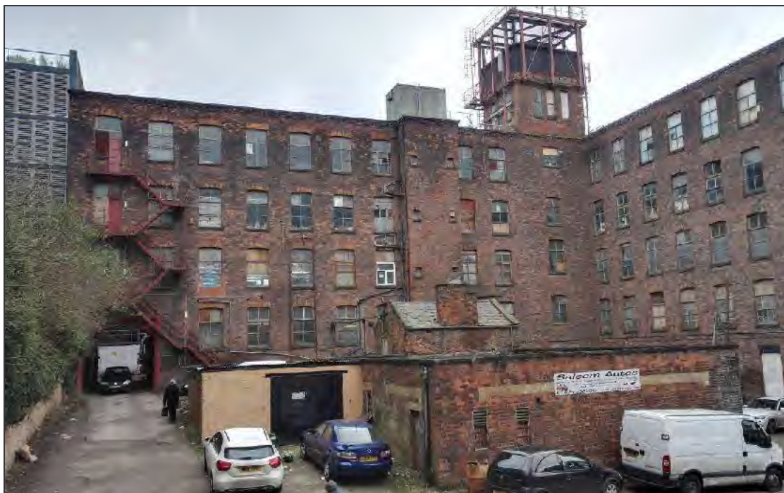
Plate 8: Mill 01 (Site 2) from the central courtyard, showing the covered entrance from Ellesmere Street
