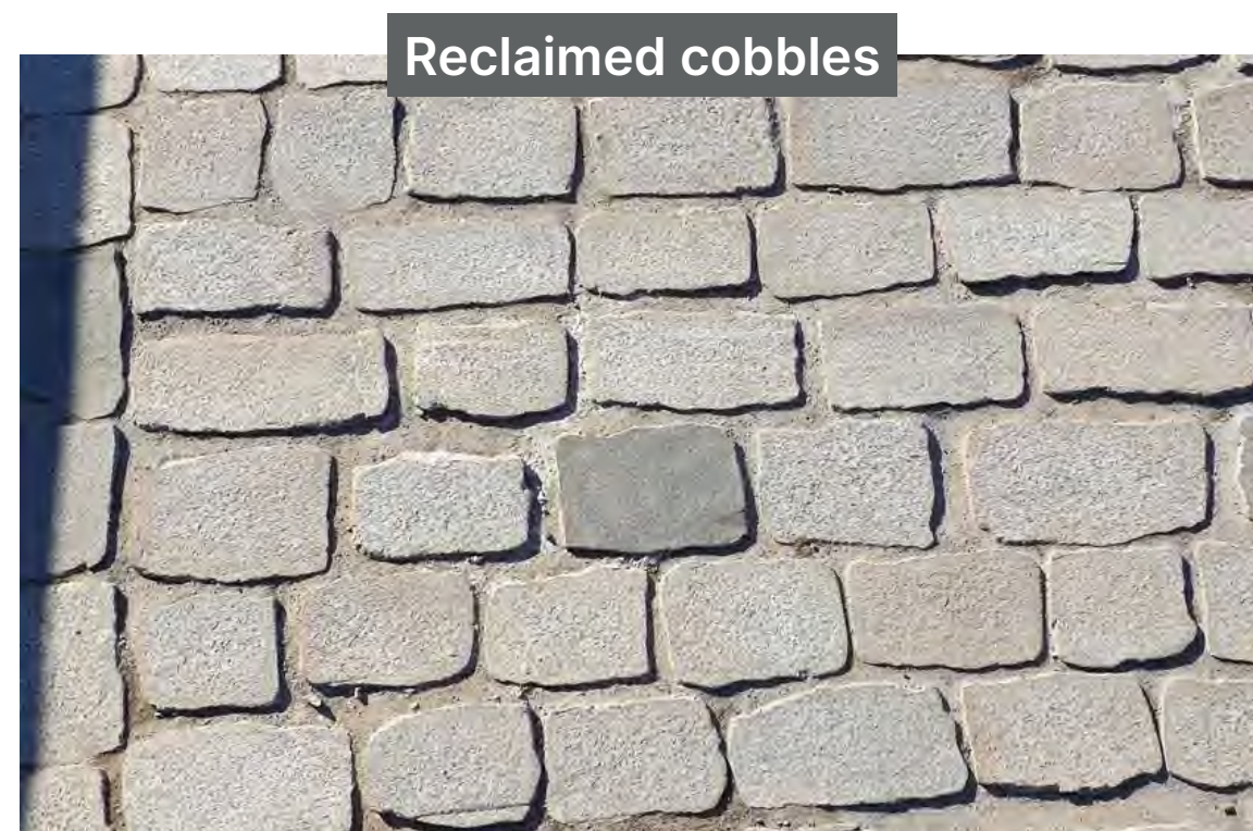
Recycled stone appearance once installed
