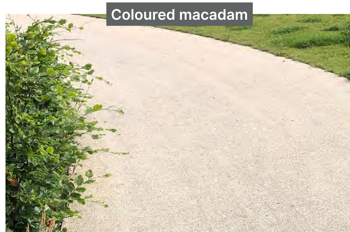
Permeable surface to allow water to drain
