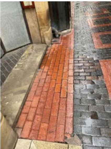
21. Change in brick type / new bricks
