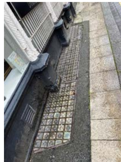
6. Overall condition of glass tiles
