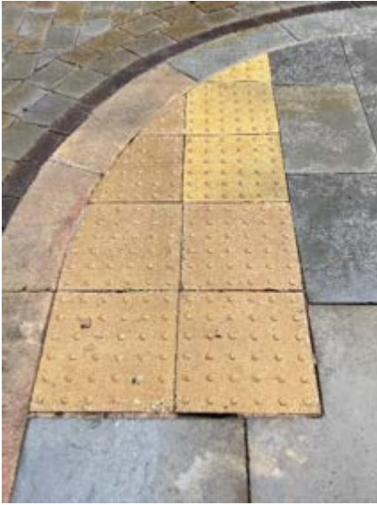
25. Missing mortar around pedestrian crossing
