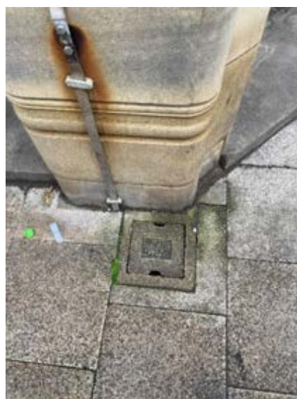
6. Earth core chamber
