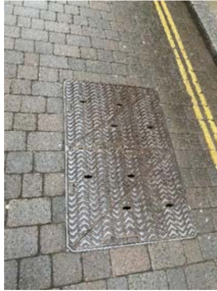
7. Partially blocked drainage inspection chamber
