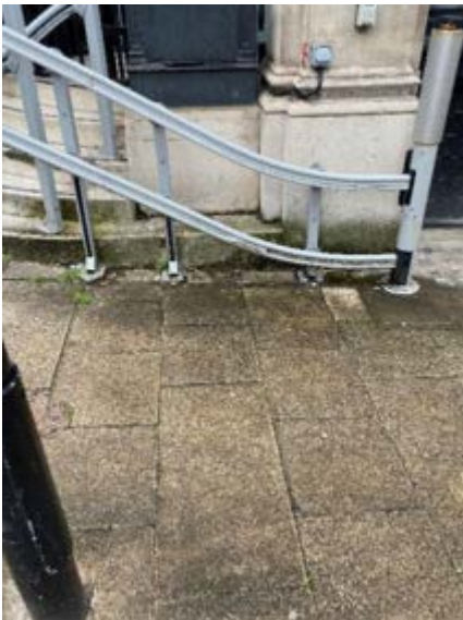
21. Stair lift condition
