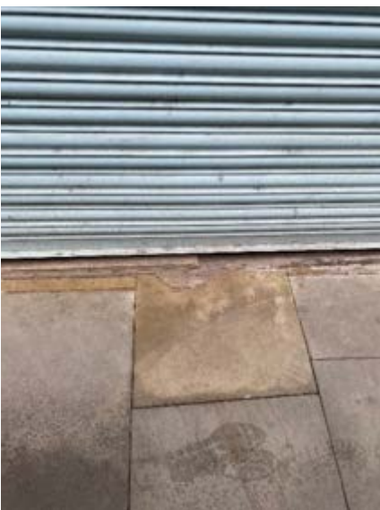
5. Raised section and concrete infill into paving
