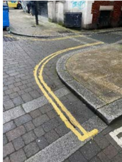
32. Repainted double yellow lines
