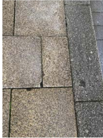
32. Chipping to tiles
