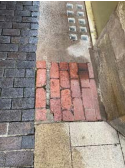
26. Concrete infill between feature bricks.
