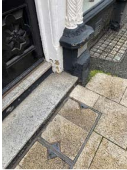
1. Some damage to tarmac & chipped tile
