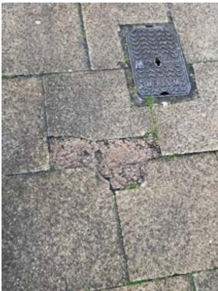
23. Concrete infill to damaged tiles
