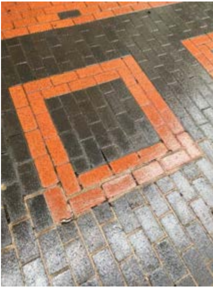
7. Replacement mortar – change in colour
