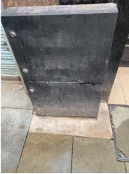
1. Service box identified, no current damage seen.
