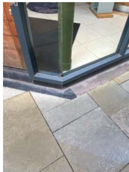
10. Continuation of tarmac infill
