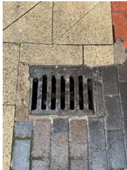
21. Change in brick type / new bricks
