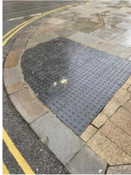
20. Pedestrian crossing condition
