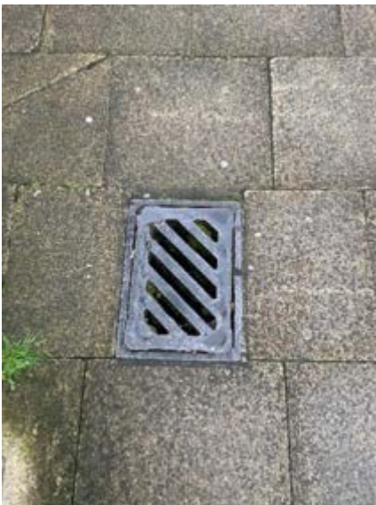
27. Clear drainage inspection chamber
