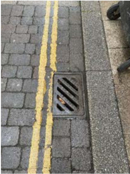
7. Partially blocked drainage inspection chamber
