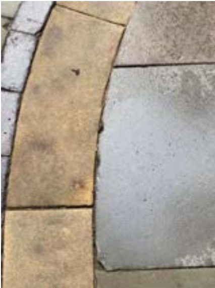
31. Chipping to paving stone
