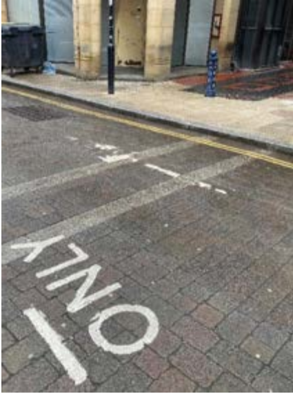
13. Arrow paint significantly faded
