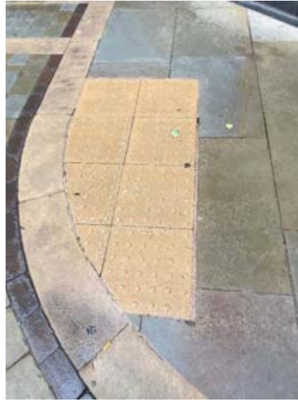
25. Missing mortar around pedestrian crossing
