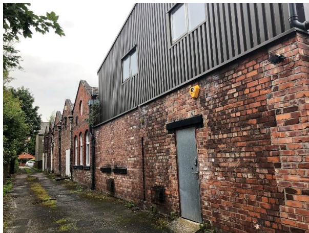
PLATE 3 SHOWING NORTH-WESTERN ASPECT OF BUILDING
