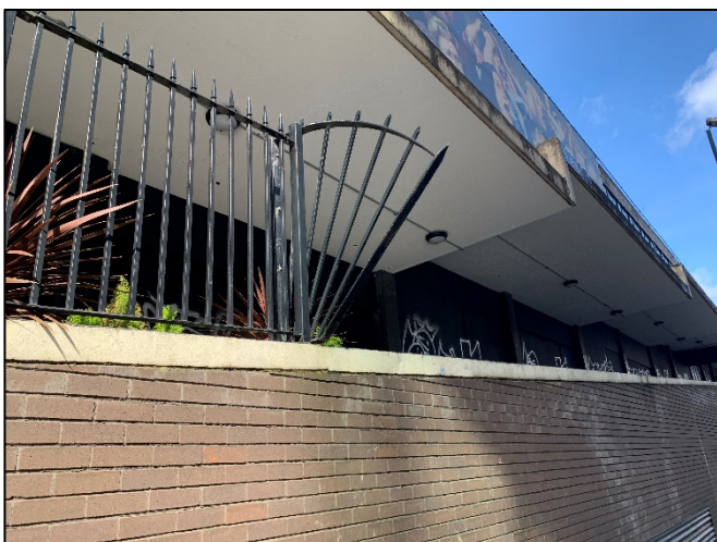
Photo 8 Eastern face retail frontage and ramp
