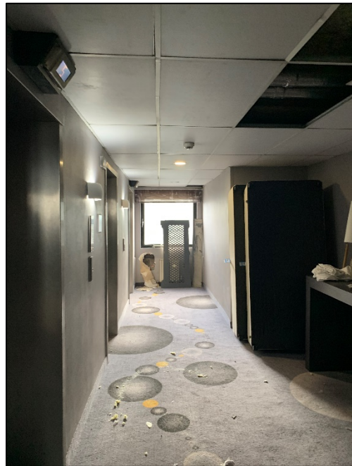
Photo 12 Example of internal aspect of the structure
