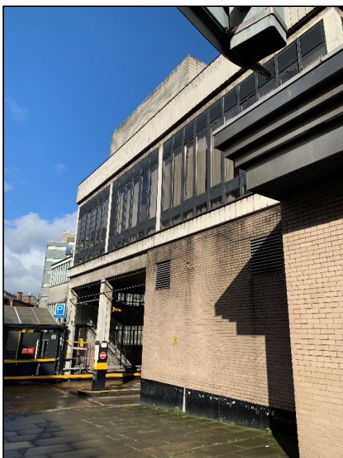
Photo 7 Southern face and entrance to NCP car park
