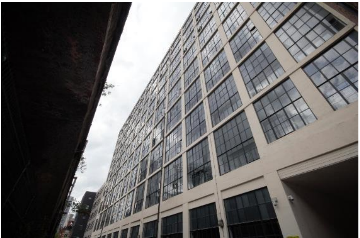
Plate 13: West elevation of Orient House demonstrating the style of the rear elements of the building.
