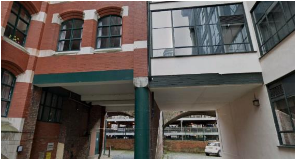
Plate 21: The covered ground floor underpasses of Granby House (left) and Orient House (right).
